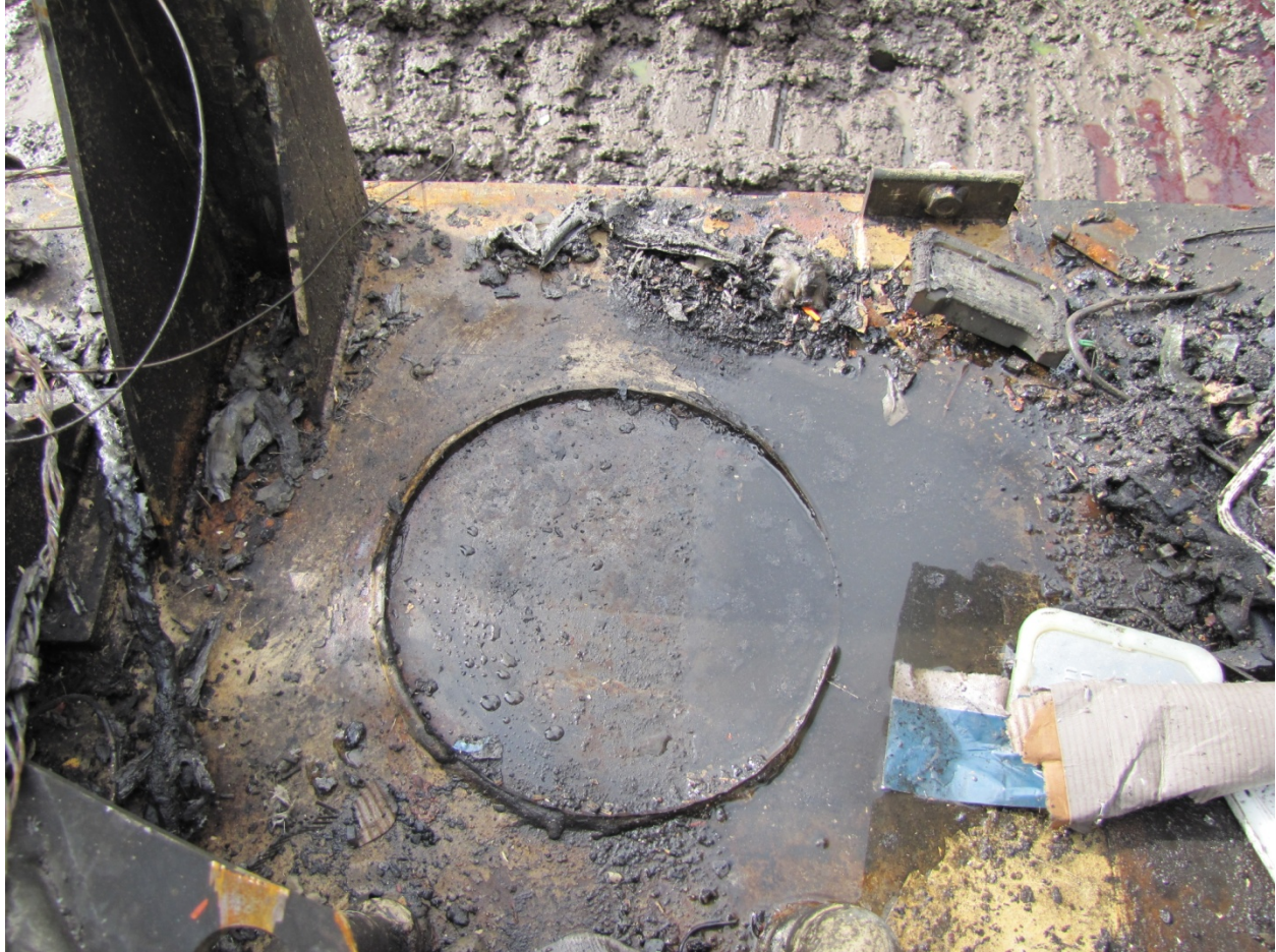
Exhibit 34- Photo Showing Broken Weld of an Operating Cab Rear Mounting Post on BNSF 9159
