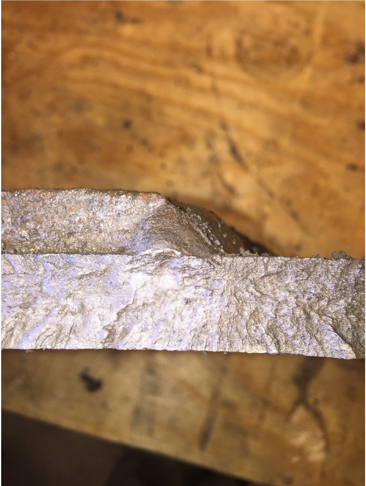
Crack initiation site and A-L cradle pad fillet weld termination
