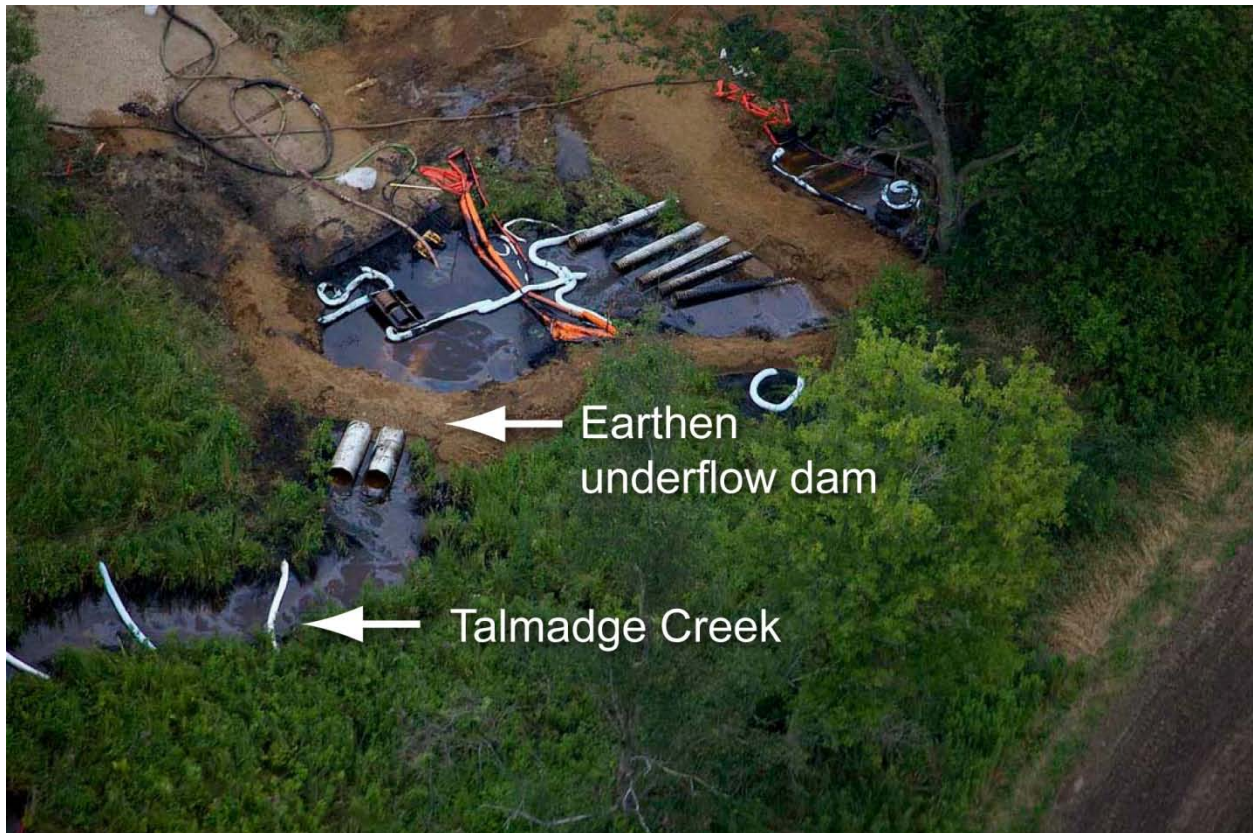
Figure 10. Underflow dam on Talmadge Creek on July 30, 2010.
