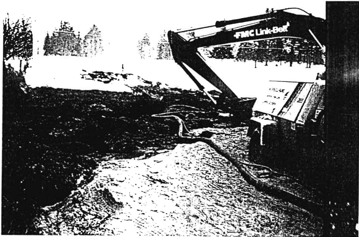
DRAIN-UP OF FAILED PIPE AND FAILURE AREA IS UNDER WAY.
