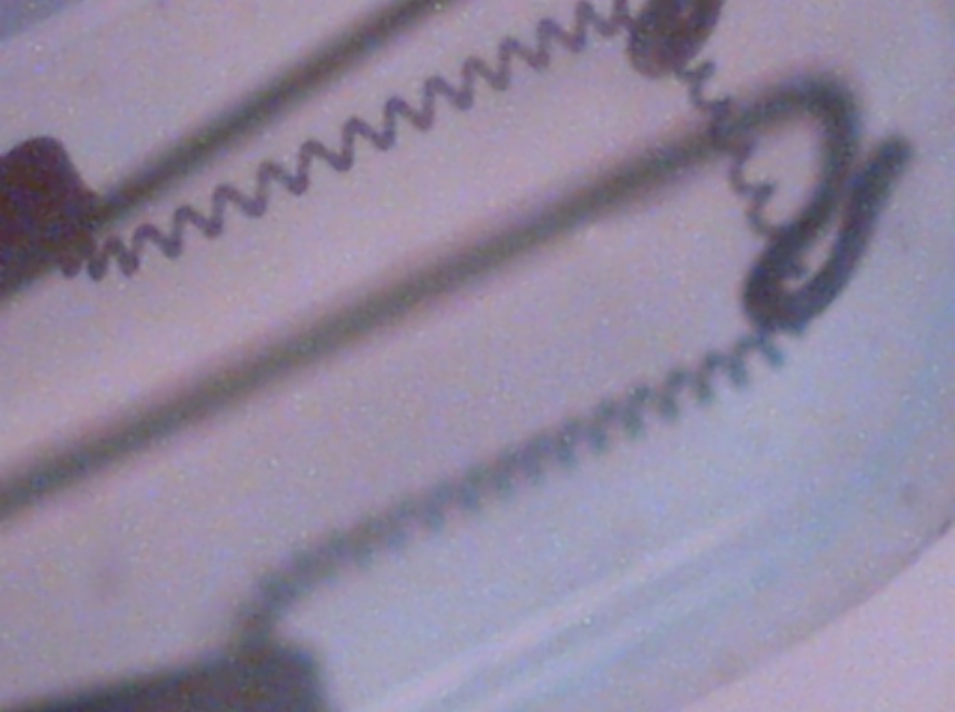
Control Panel Photo 7 - Ext Pwr Bat - Bulb A
