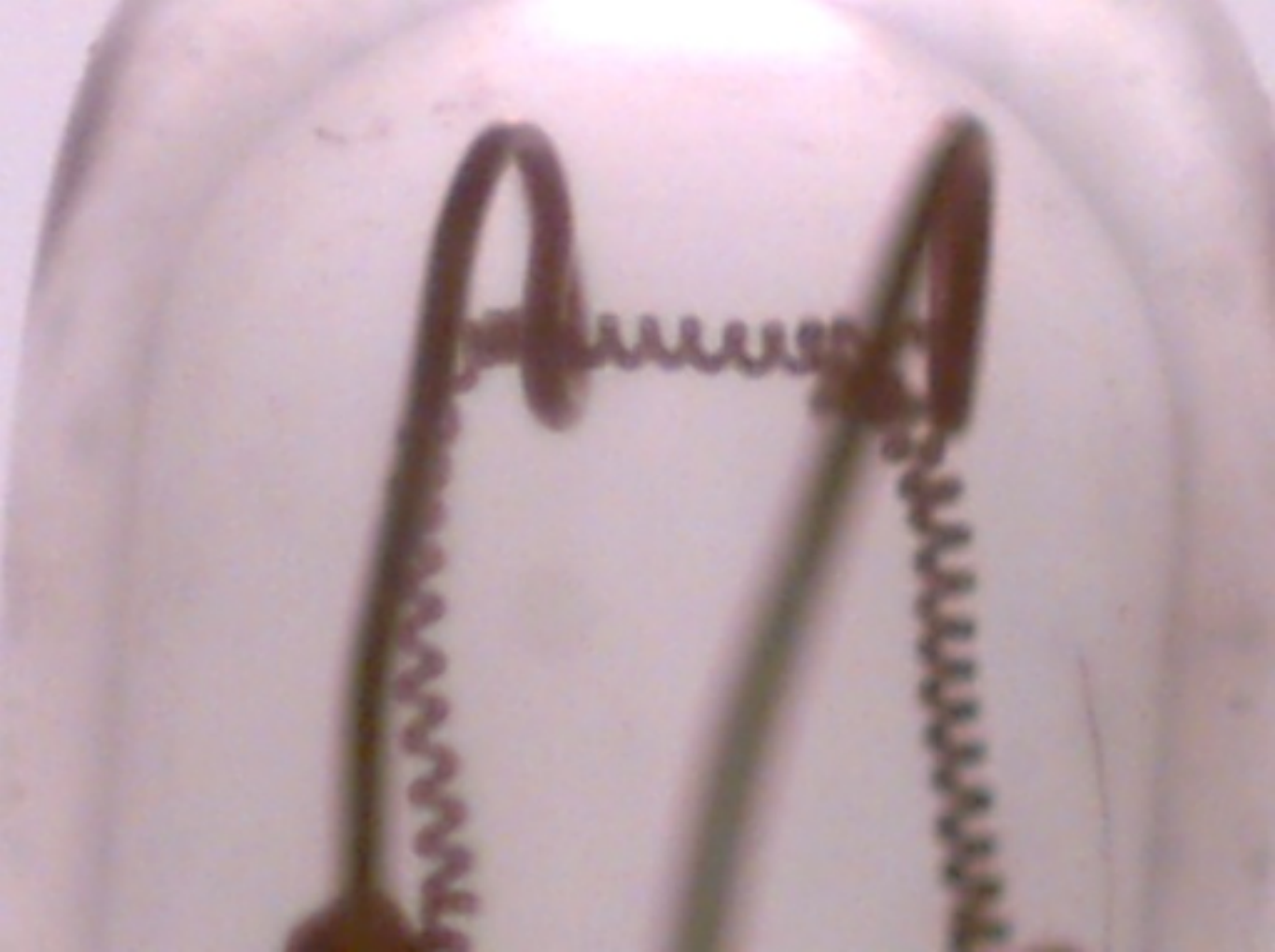
Control Panel Photo 20 - Gen - Bulb B View 2
