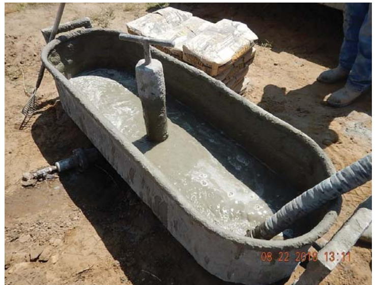
Well casing being cemented from approximately 79' in depth to 6' below grade
