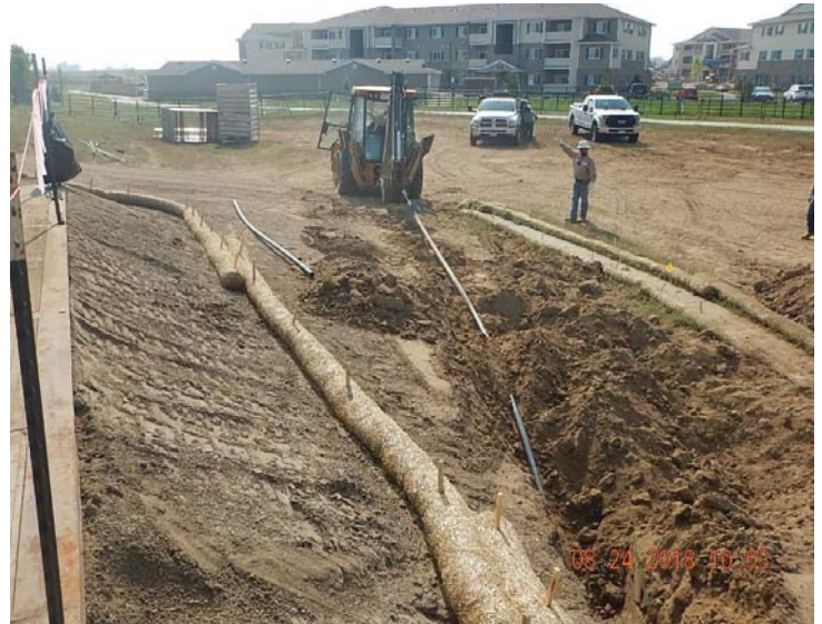
Final segment of flowline from Coors V 6-14 removed near well (now PA).
