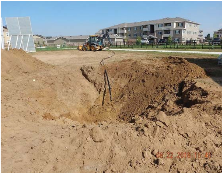
Flowline being removed at Coors V 6-14JI (PA) wellhead
