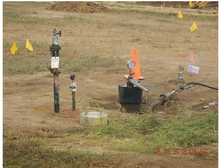
View of Coors V 6-14 JI well casing being pressure tested
