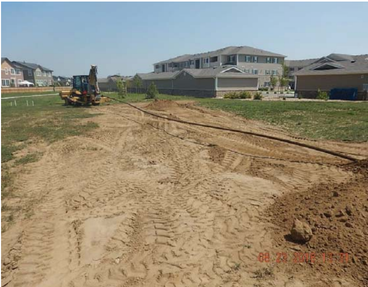
Flowline removal in progress (Coors V 6-13) east of Oak Meadows Blvd.
