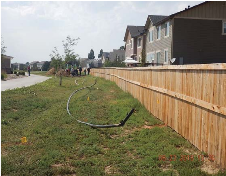
Flowline removed from ROW south of Oak Meadows Subdivision from Coors V 6-14JI (PA) well
