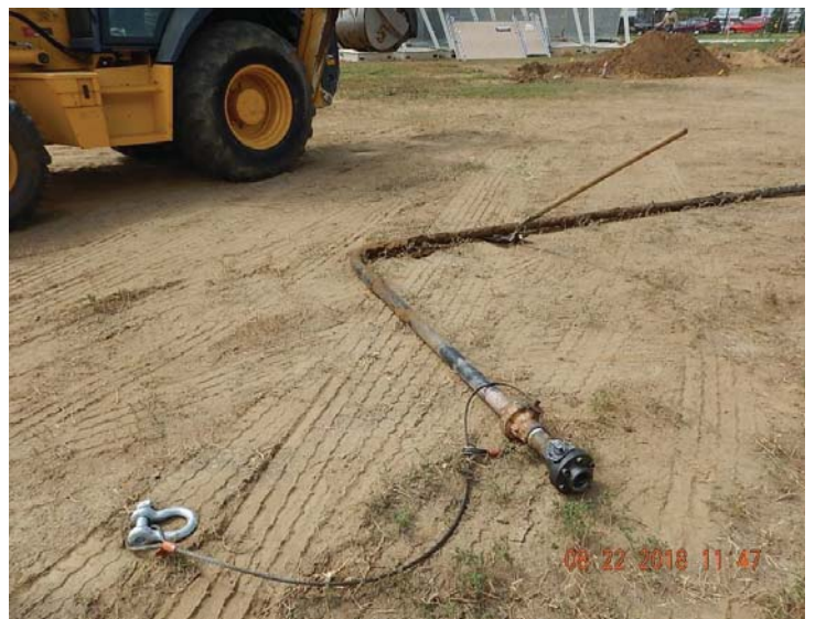
Flowline risers excavated and removed at Coors V 6-14JI wellhead/ location
