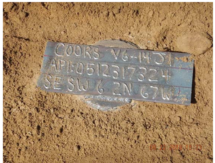
Welded cap on Coors V 6-14JI well casing (PA) to be backfilled and buried 6' below grade
