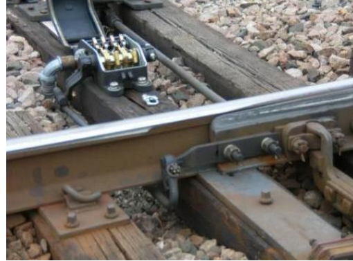
Figure 2. Apparatus at the Switch
