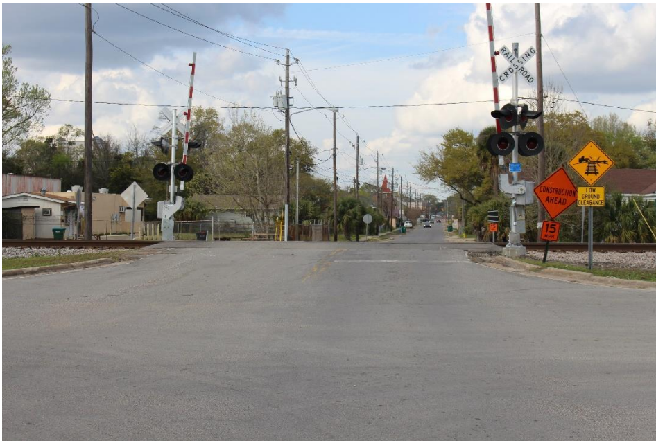
Figure 1. Northbound view of the highway-rail grade crossing at the crash site.
