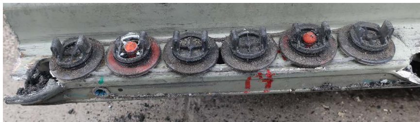
Figure 49. Module 14 valves after removal.
