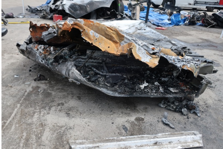
Figure 40. View from front into exposed and empty modules 15 and 16.
