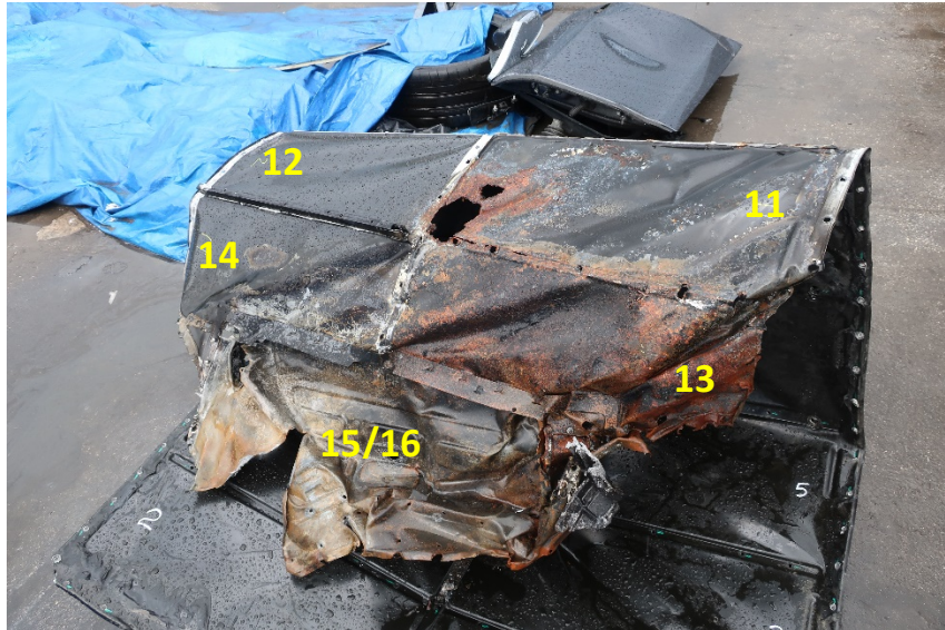
Figure 65. The inside surface of the top steel battery cover has a set of holes over where the forward terminal had been for module 11. Numbers have been added to denote modules.
