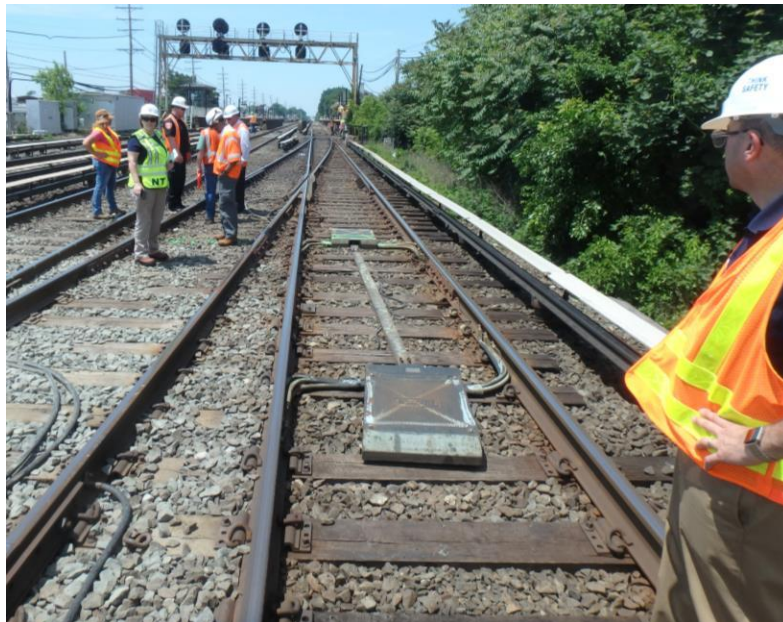
Figure 1. See photo below of approximate location of where Foreman was struck (MP 13.3):
