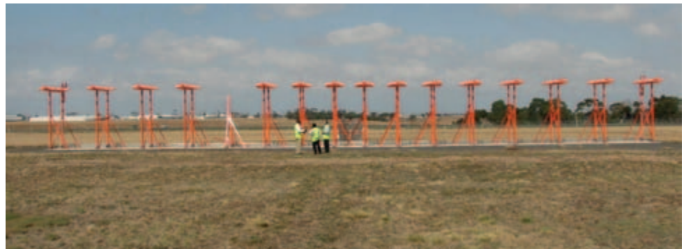
Figure 3 ...and to a collision with a runway light.
