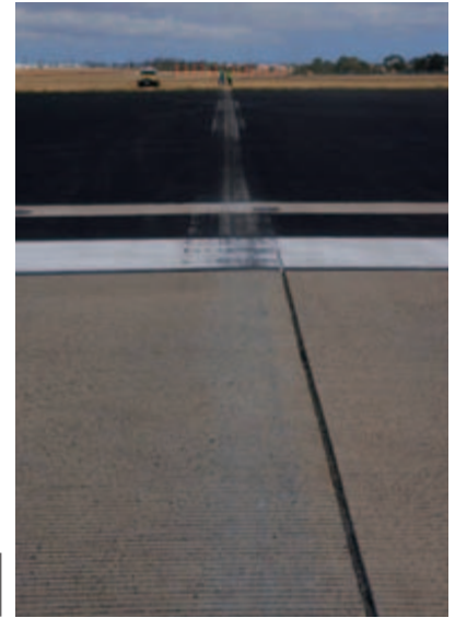
Figure 2 Entry of a gross weight lower than the actual aircraft weight led to a tailsrape...
