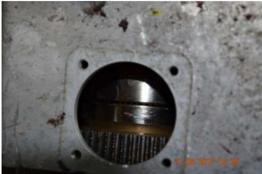
View through inspection plate of main drive gear.
