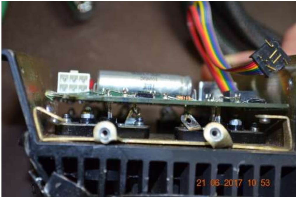
KTA 336 SN 1794 Interior view 3.
