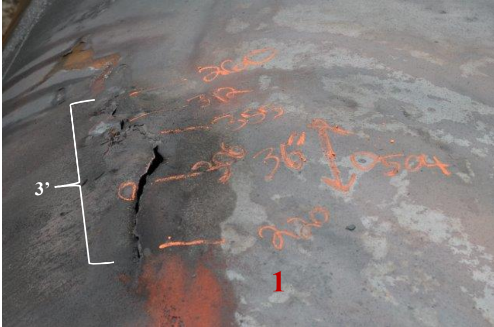
Figure 23: Thermal tear CBTX 741926 showing shell thickness measurements.
