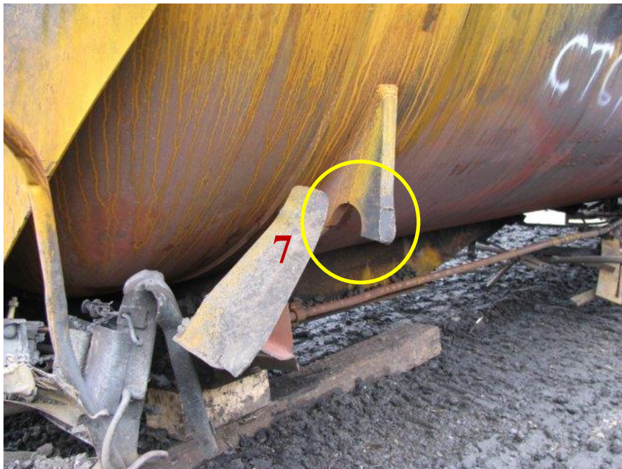
Figure 38: Upper bolster structure protuberance after bottom structure torn away at B-R end.
