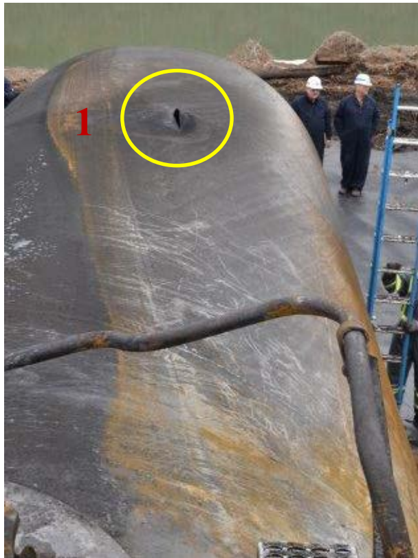
Figure 11: GATX 286232 thermal tear.
