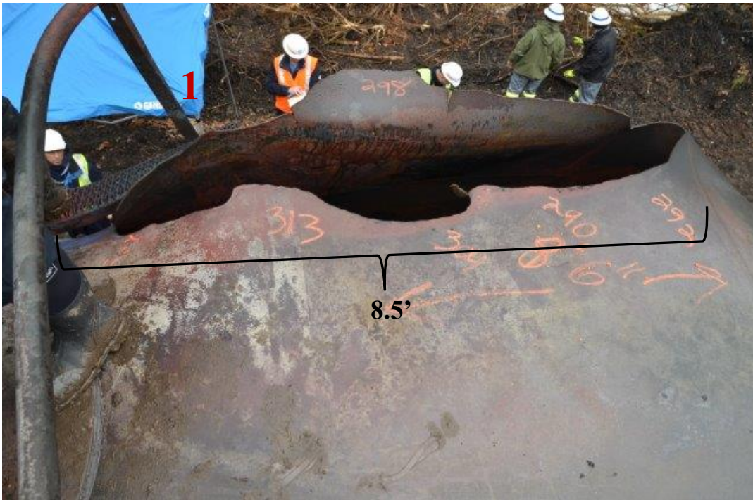
Figure 16: GATX 286292 thermal tear with steel thickness measurements.
