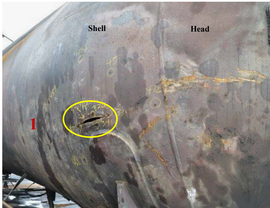
Figure 63: CBTX 742087 thermal tear above bolster pad (circled).
