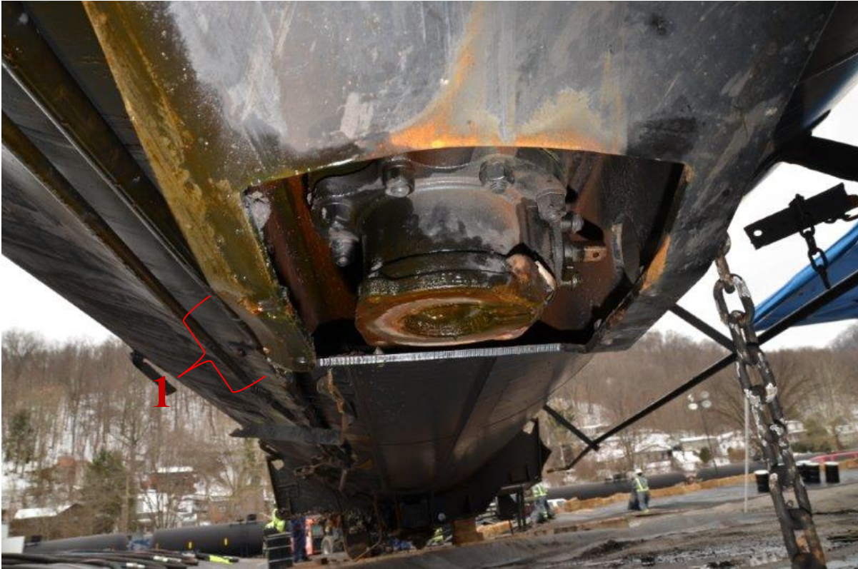
Figure 5: GATX 286233 bent skid protection indicated by Item 1, and leaking bottom outlet valve.
