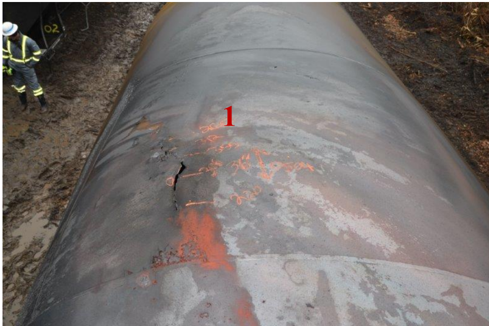
Figure 24: Thermal tear as seen from top of car looking toward B end.
