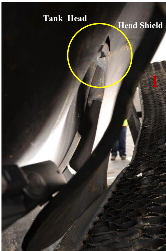
Figure 70: View between A-end head shield and tank head showing fractured head shield and impact damage to tank head (circle).
