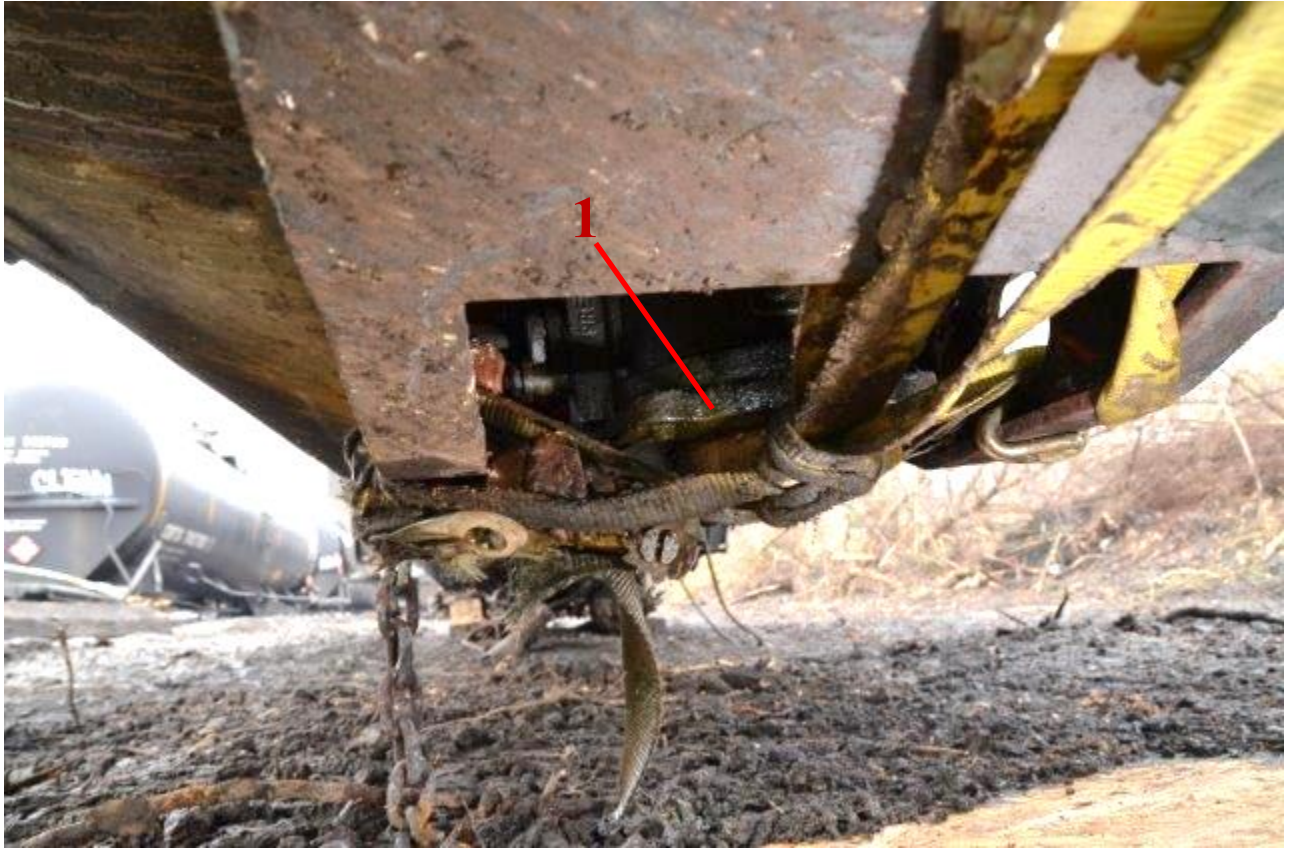
Figure 19: GATX 286274 bottom outlet valve fitted with wooden plug and straps to secure leakage.
