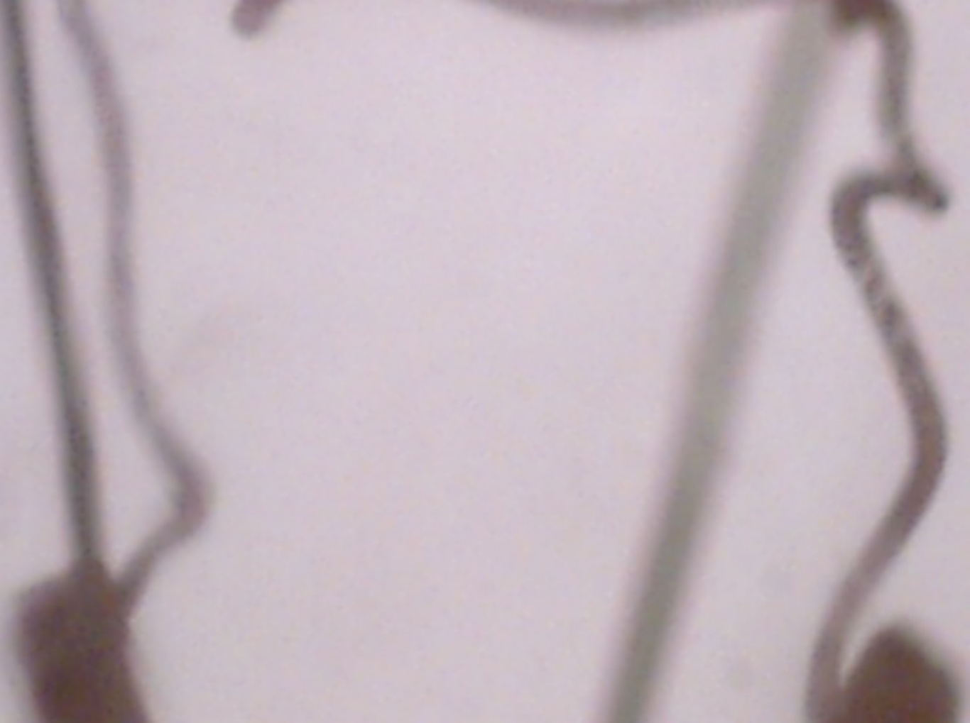
Annunciator Panel Photo 38 - Fire - Bulb A View 3
