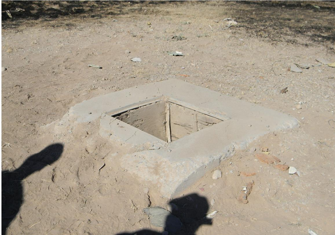
Figure 10 Concrete Culvert for Electrical Access
