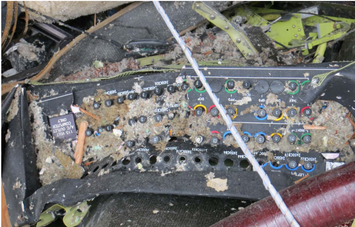
Figure 1 - Co-Pilot's Circuit Breaker Panel at Accident Site
