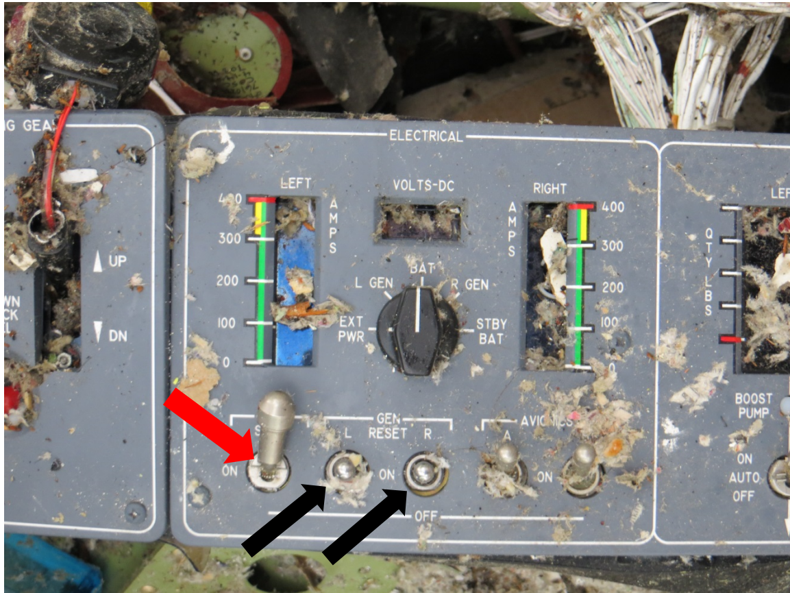
Figure 2 - Electrical Panel, Including L and R GEN Switches (black arrows) and Standby Battery Switch (red arrow). (Note: Photograph taken at accident site)
