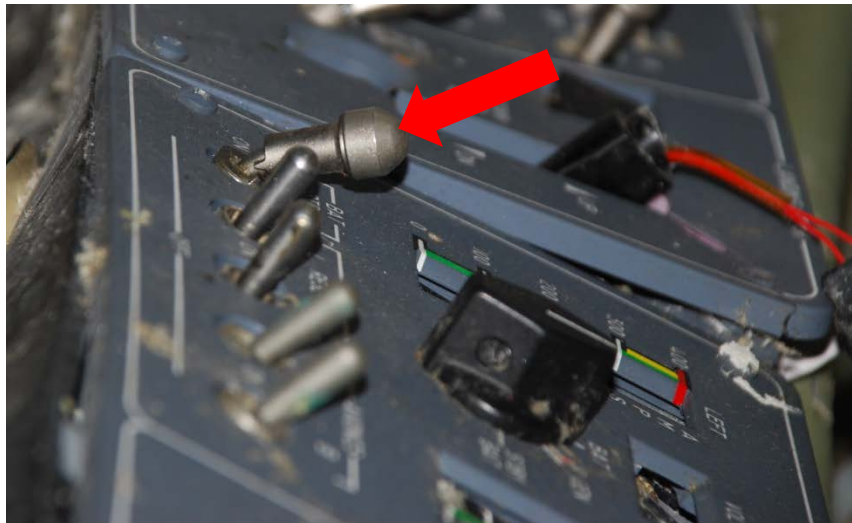
Figure 3 - Standby Battery Switch, After Wreckage Moved to Hangar
