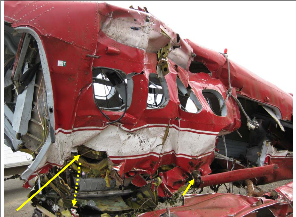
Figure 20. Damage to left side of the cabin. Arrows point to the approximate displacement of the left float fittings. The aft edge of the cockpit door is normally vertical (above long arrow) and the crush aft of it is how far aft the cockpit/cabin bulkhead had been displaced toward the cabin's left forward-most seat. The seat had been above the head of the long arrow. (As the fuselage was lifted, the forward bulkhead remnant and left forward float attachment fell to the end of the dashed line.) Also visible above the windows is the amount of intrusion into the upper fuselage by the trailing edge of the left wing.
