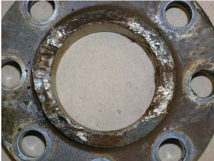
Photo No. 62 Propeller mounting flange, detail.
