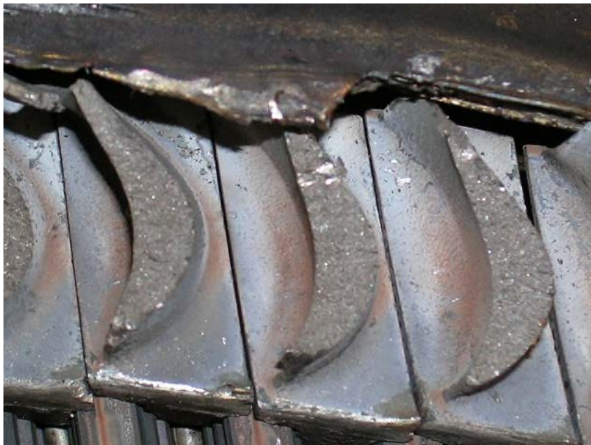
Photo No. 52 Power turbine blade roots, detail
