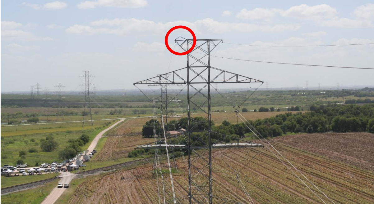
Figure 5 - Bent elbow on Tower Structure 127 (circled). Transmission T511 lines are on left side of tower, Transmission T510 lines are on right side of tower.
