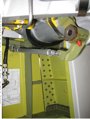
Figure 38C. Learjet Model 45 at top of right main landing gear strut, forward of the photo above (Figure 38A) and above the inboard tire plane of rotation.
