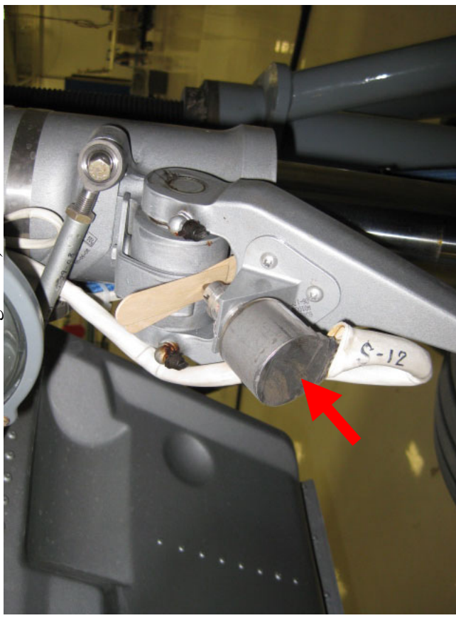
Figure 37B. Learjet Model 60 with an arrow indicating the single exposed squat switch on right main landing gear. (The photo includes a wooden stick that was installed to simulate air mode during tests.)
