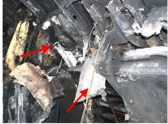
Figure 38 N799AX: The top of the L1 door, with the upper arrow pointing to the remaining end of the door track and the lower arrow pointing to the slack counterbalance cable.
