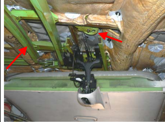
Figure 37. Exemplar airplane: Photograph of the door when raised to the top of the tracks. The left arrow points to a track and the right arrow points to the counterbalance pulley.
