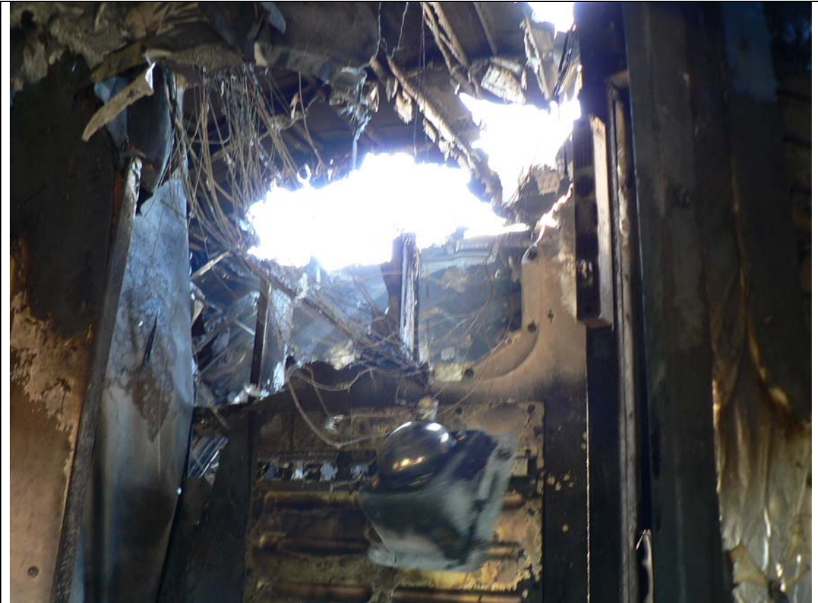
Figure 5. As viewed aft and up from the Captain's seat in N799AX, this view shows where fire breached the wall that had separated the cockpit from the supernumerary compartment. The sky is visible through the holes that had penetrated the top of the supernumerary compartment. The supplemental oxygen tubing and wiring that were not found for inspection had been in this missing area.
