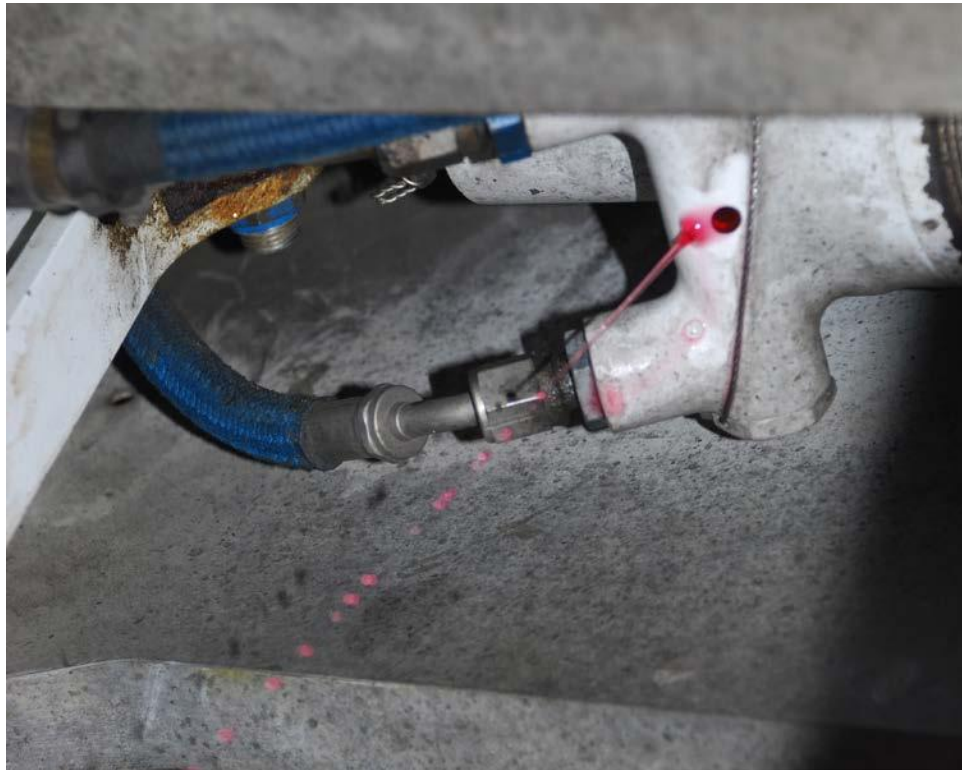
Figure 5 – LMLG Actuator Leak
