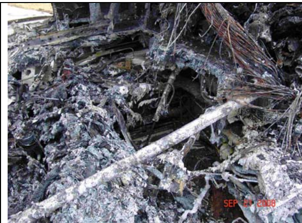
Figure 17. The right main landing gear well from above right, as exposed by the post-crash fire.
