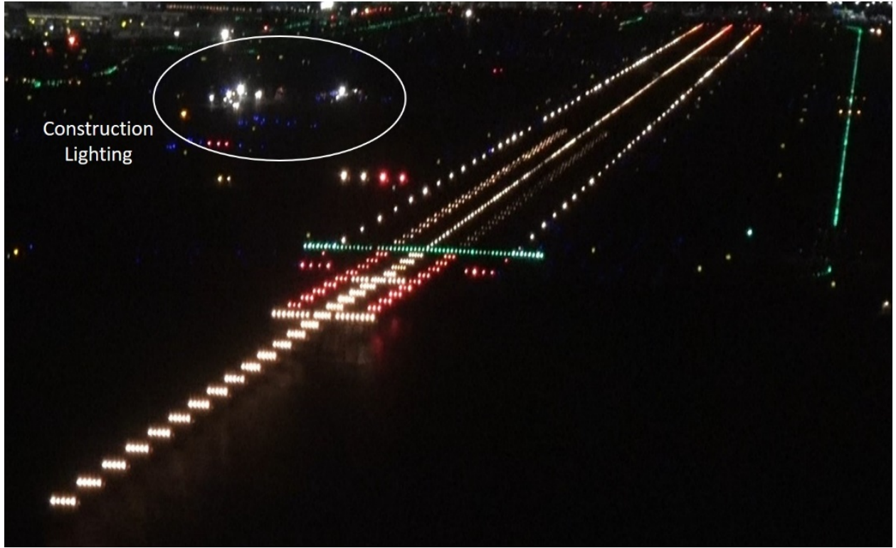
Photograph 4 – Construction Zone on runway 28L.
