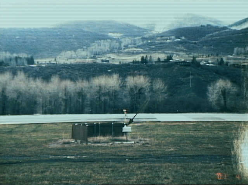
Airports/ARFF 16 - Attachment 3 - Photo 1. A view looking 060 degrees magnetic along the threshold lights showing the right REIL unit (arrow depicts lamp) and flash shielding northwest, northeast and east.
