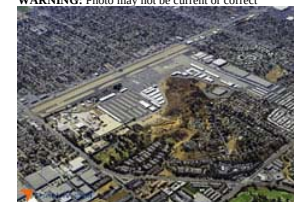
Photo by Zoltan Szalva Photo taken 23-Sep-2010 looking west.
