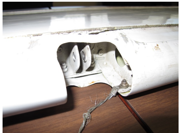
Left elevator - inboard hinge point.
