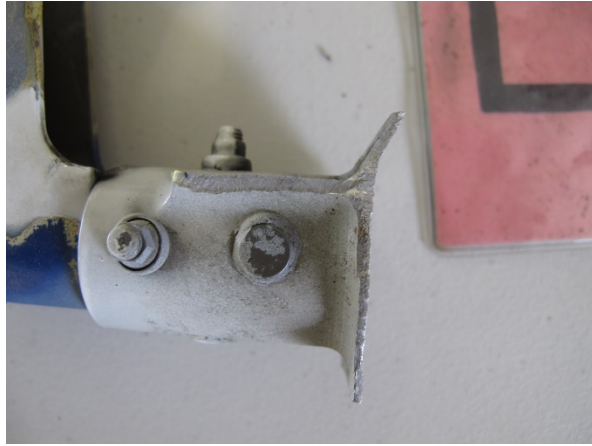
Left elevator command lever torque tube fracture.
