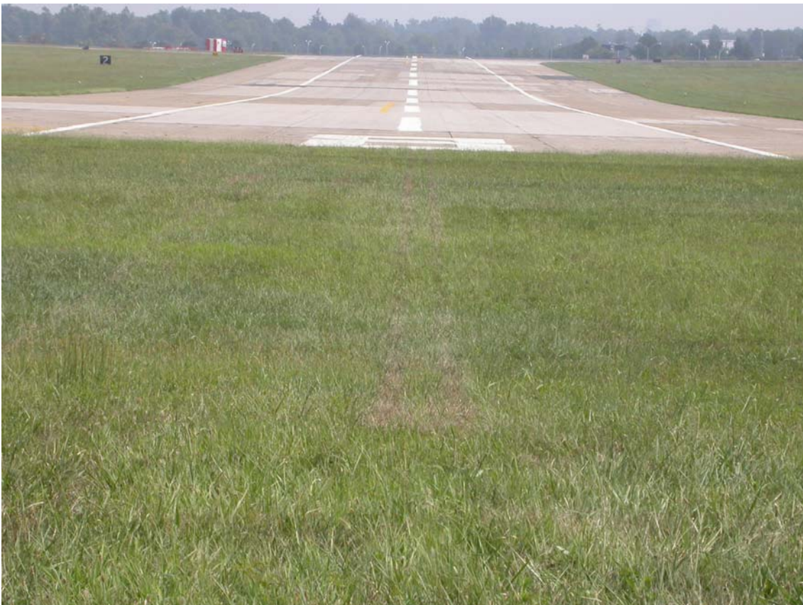
Figure 1: Departure End of Runway 26 Looking Back Towards the East
