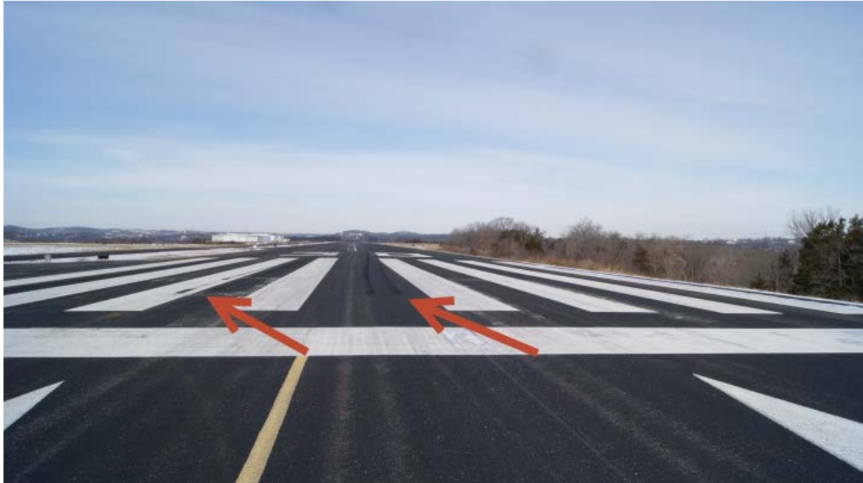
Figure 5 – The departure end of runway 12/approach end of runway 30 at PLK. SWA4013 main mount tire tread marks are indicated by red arrows.
