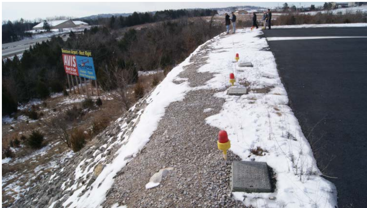
Figure 4 – The approach end of runway 30/departure end of runway 12 facing southwest
