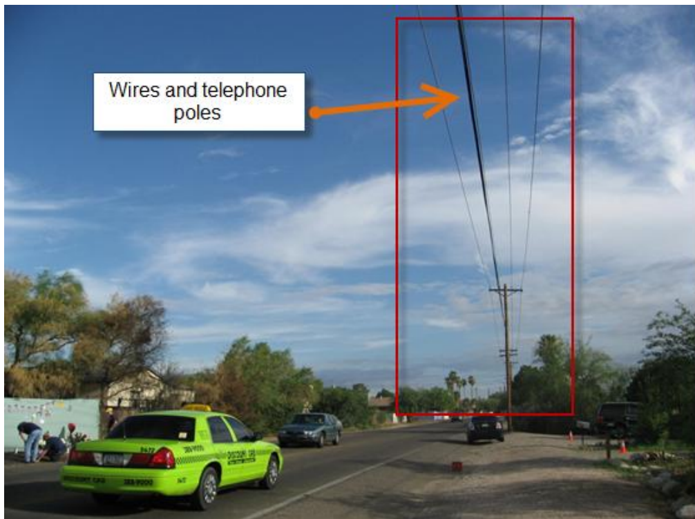
Photo 6 wires on west side of street
