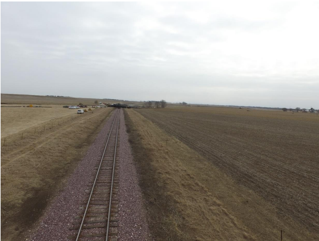
Figure 8 – Segment of track approaching site along direction of travel
