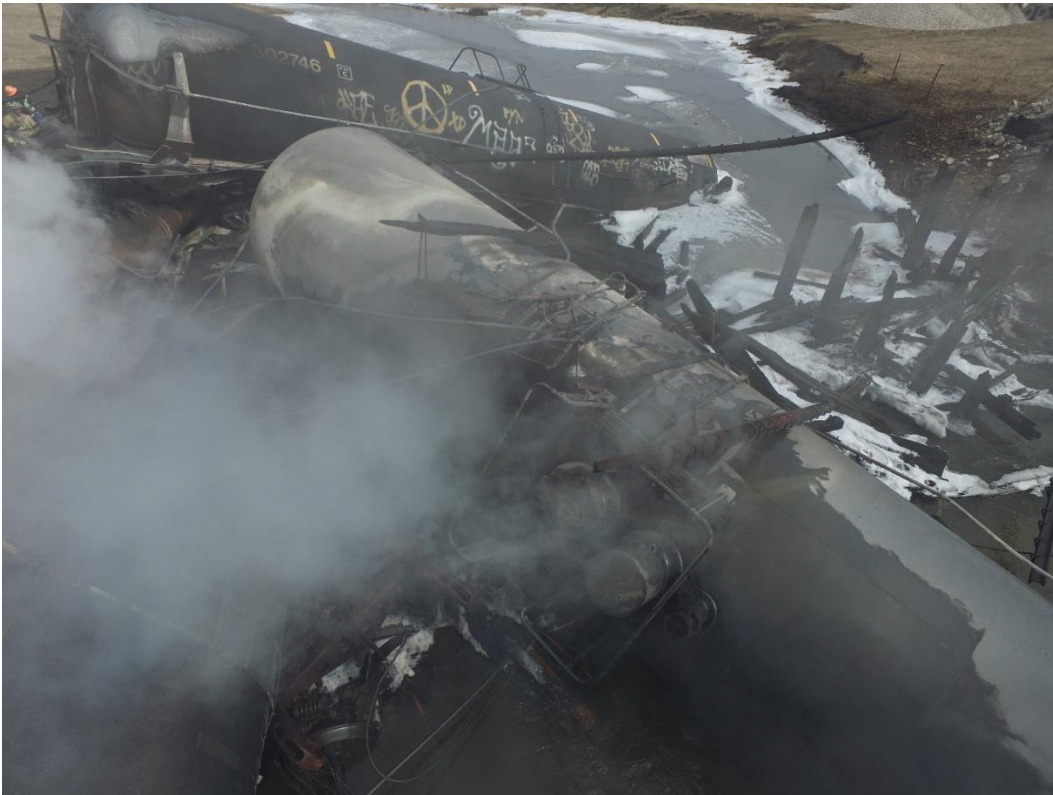
Figure 7 - Trestle and fractured track from west side
