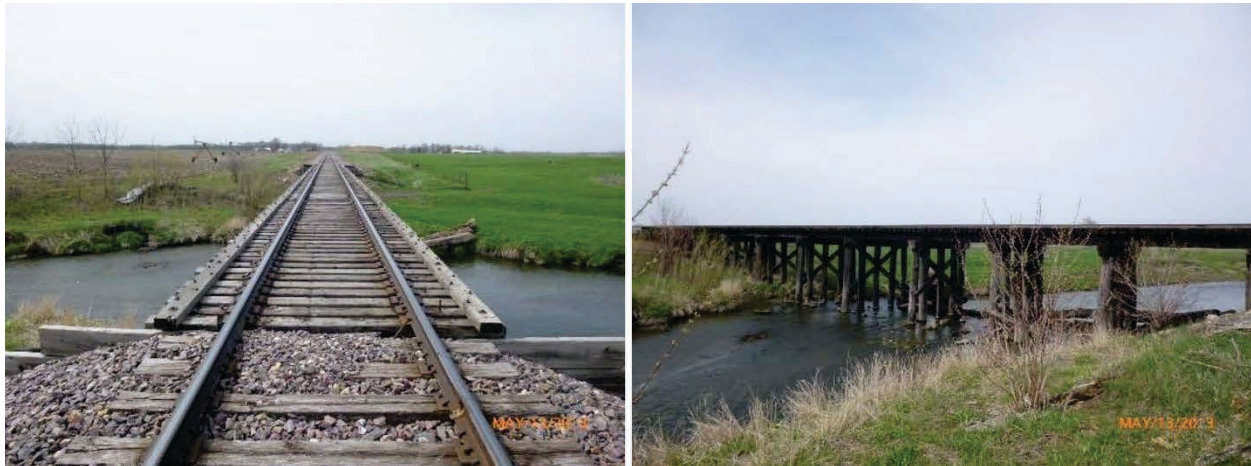
Figure 8. Jack Creek Bridge in 2013. (Photographs courtesy of UP.)
