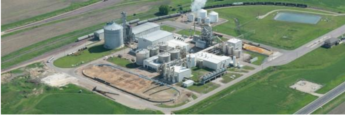
Figure 2. Green Plains ethanol facility in Superior, Iowa. (Photograph courtesy of the Green Plains website.)
