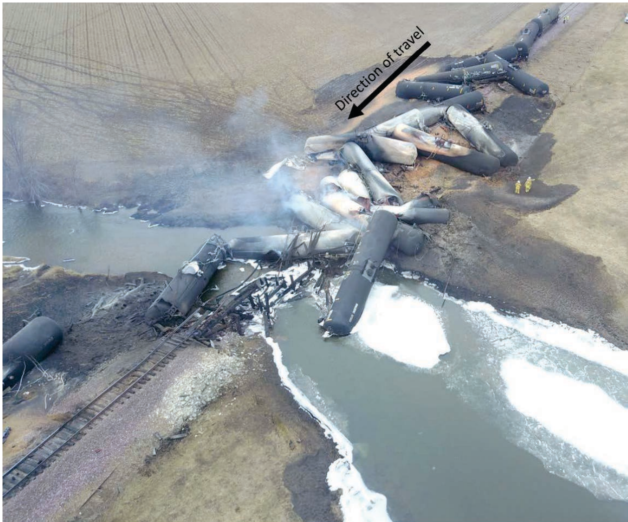
Figure 6. Aerial photograph of the derailed train and the damaged track.
