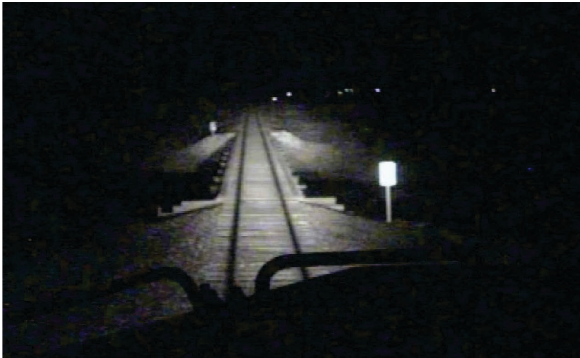
Figure 9. Still image of the track on approach to the Jack Creek Bridge.
