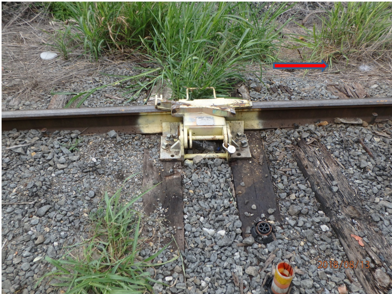
Figure 3. Photo of derail on track 400 and location of conductor's switch keys.
