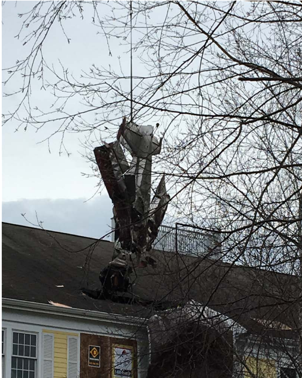
Photo 4 – View of airplane recovery from roof of condominium.
