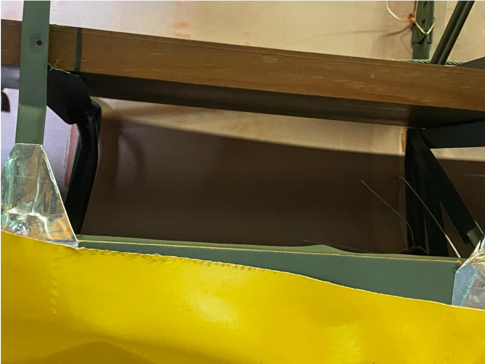
Photo 5 – No damage to right wing main spar (FAA photo)
