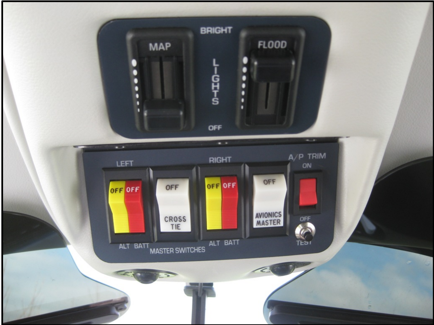
Photo 8 – Master Switch Control Panel (FAA Photo)
