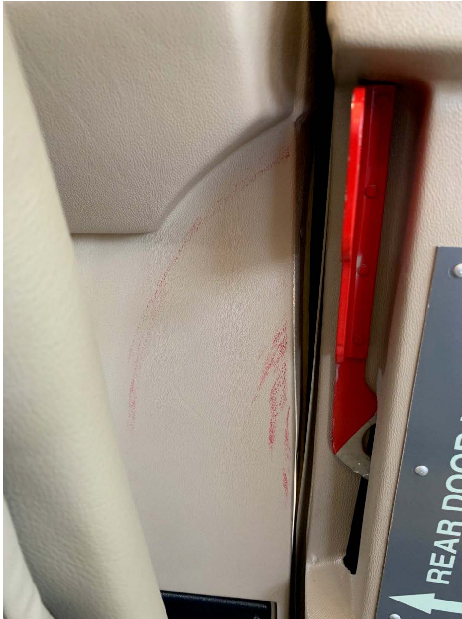
Photo 2 – View of right rear passenger door latch in up/closed position (Photo courtesy of the FAA)
