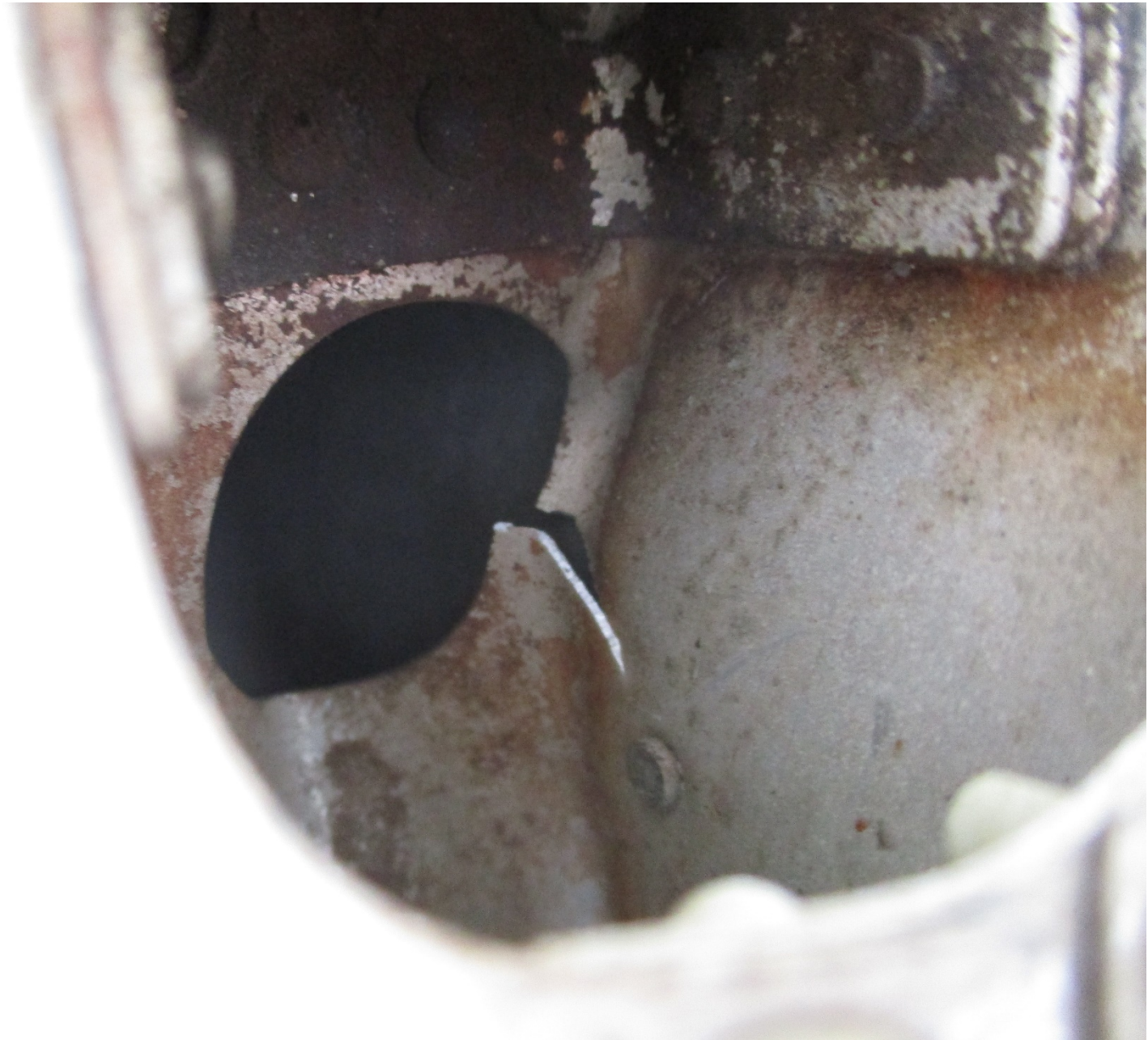
Photo 2 – View of internal rudder damage of N704VM (Photo courtesy of the student pilot)
