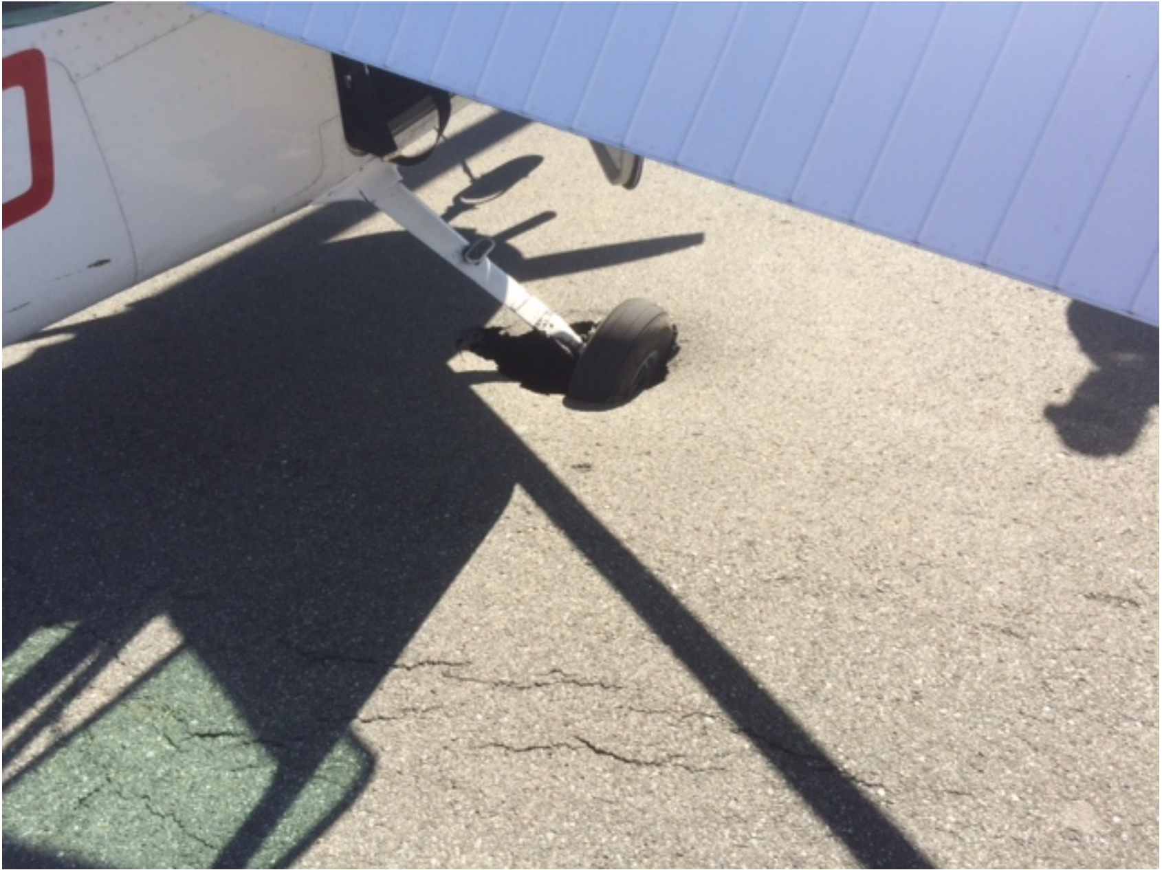
Photo 2 - View of right main landing gear in sink hole (photo courtesy of the FAA)
