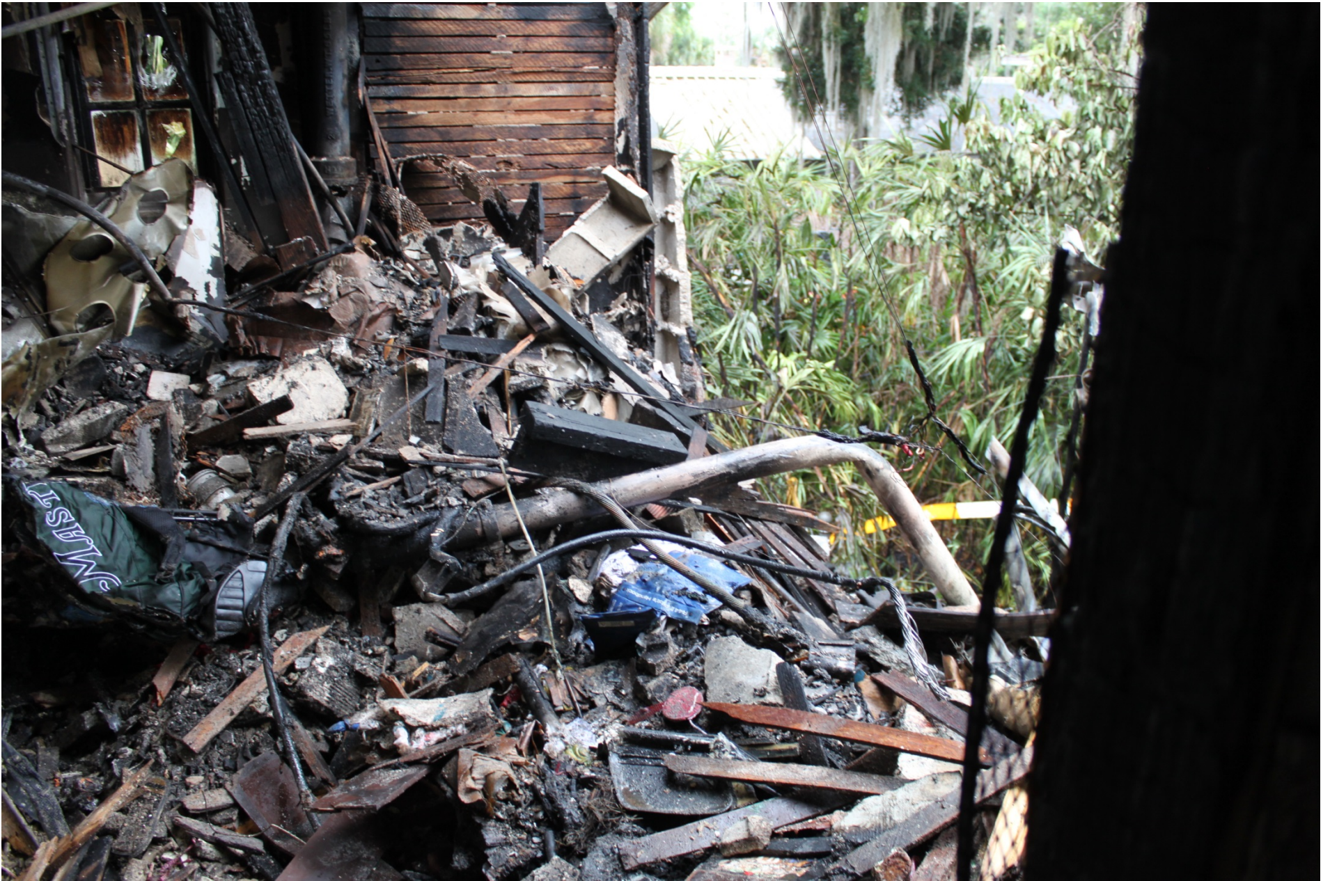
Photo 1 –View of main wreckage
