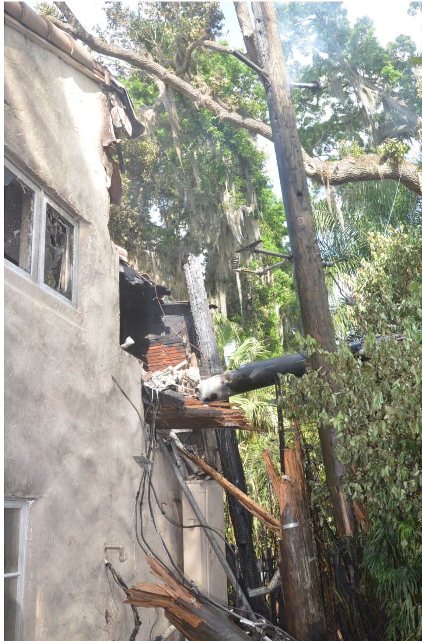
Photo 20 –View of accident site
