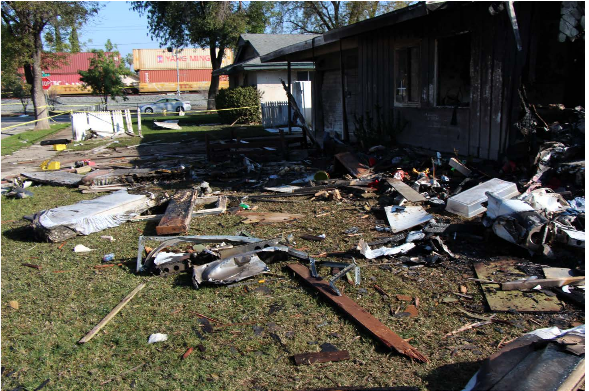
Photo 4 – Debris Path Beyond the Main Wreckage
