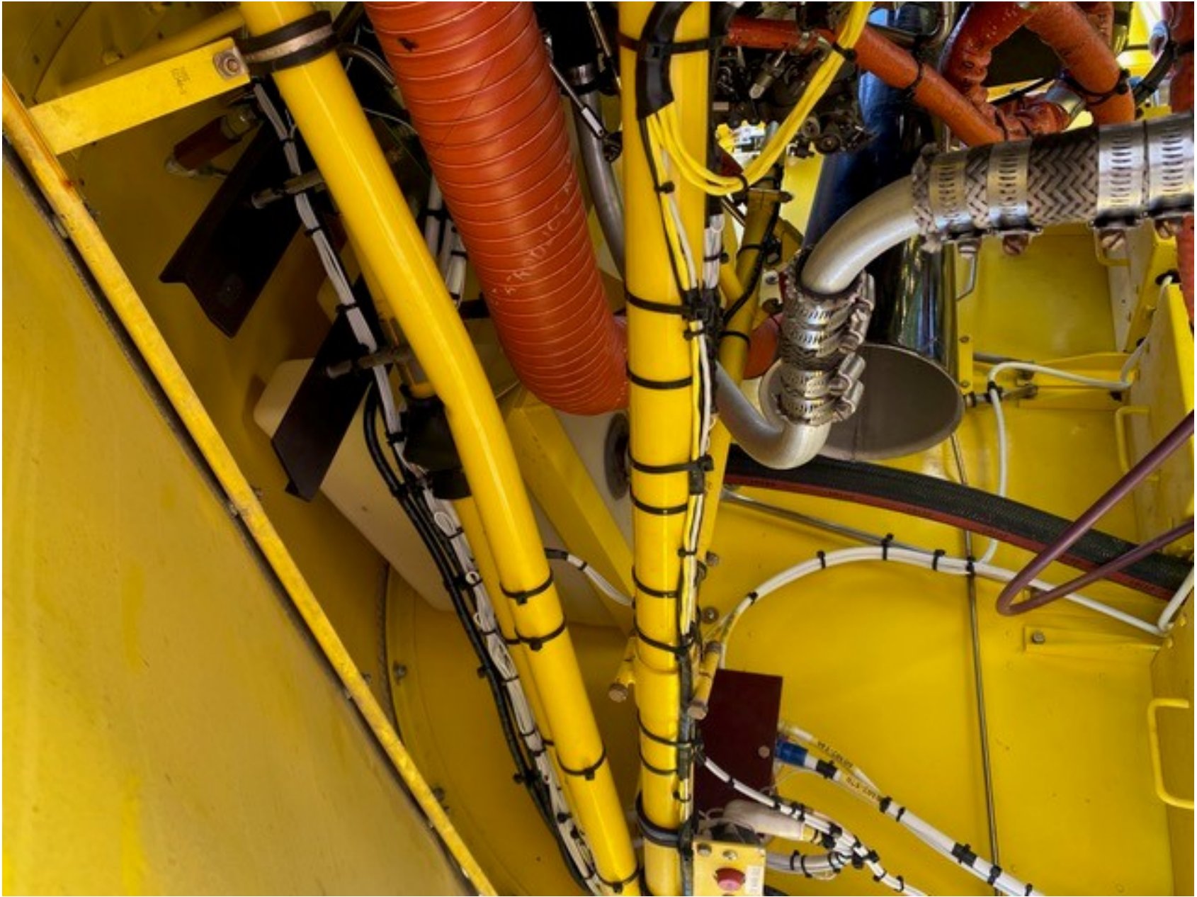
Photo 5 – View of the damaged engine mount (courtesy of Lane Aviation, Inc.).
