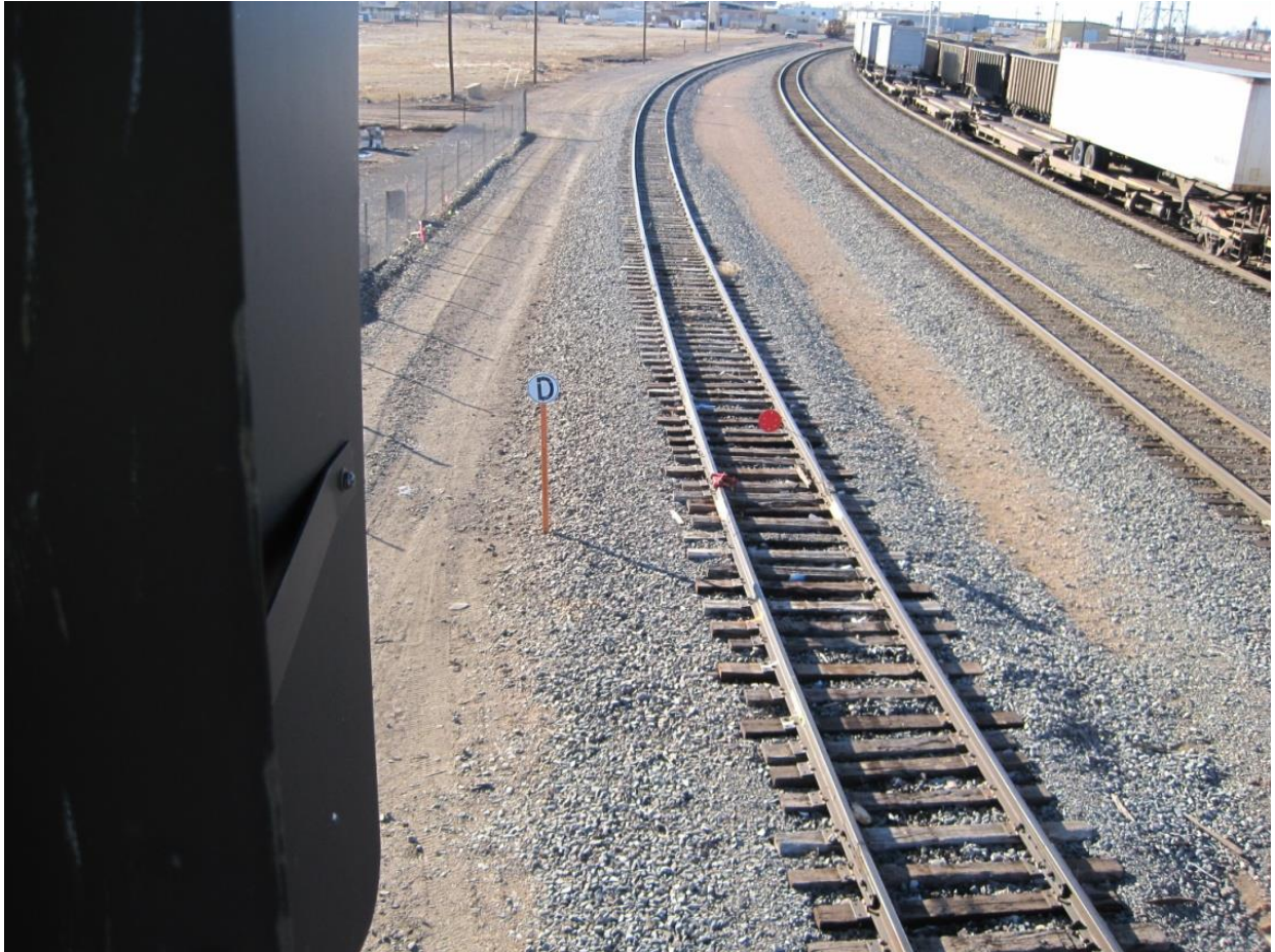
Figure 3. Overhead view facing west of track No. 1805 with derail opposite signpost D.
