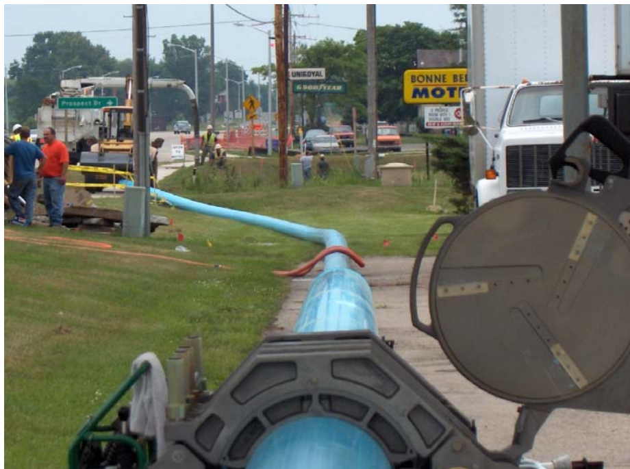
Figure 4.6 – Pipe Bursting with PVC Pipe
