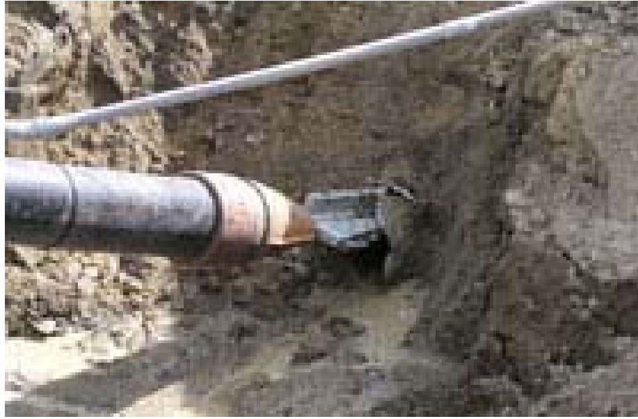
Figure 4.5 – Pipe Bursting with HDPE Pipe
