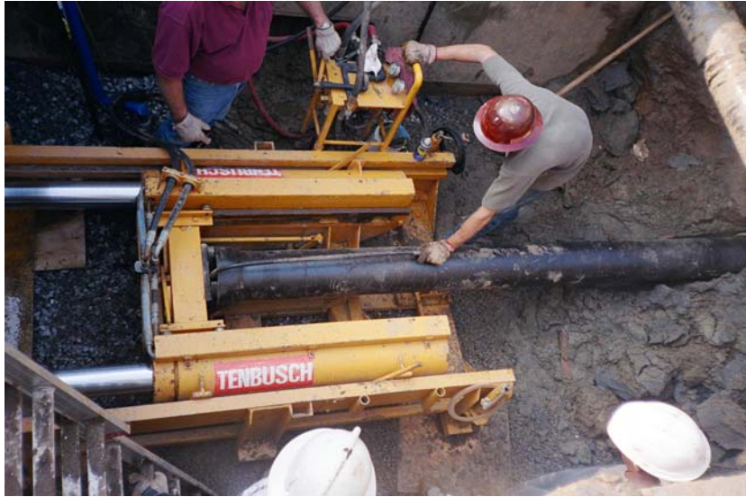
Figure 4.4 – Pipe Bursting with Ductile Iron Pipe
