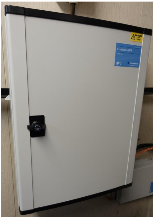
Figure 5. Consilium VDR main unit, exterior
