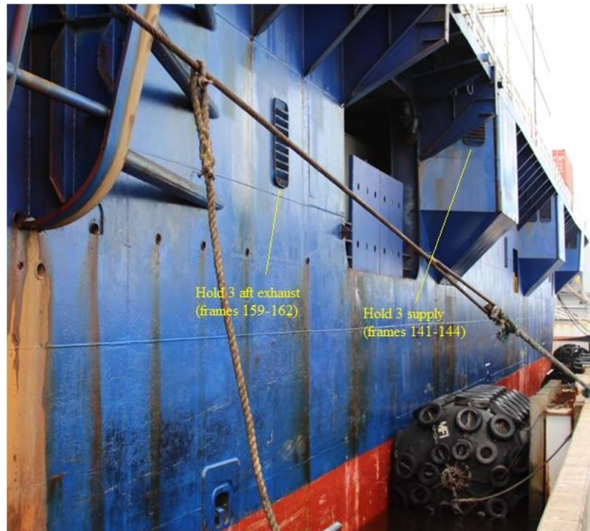
Figure 6-10: Starboard ventilation louvered hull openings for Hold 3 ventilation supply and aft exhaust. Note that red paint delineates the load line (approximate full load waterline). Photo of sister vessel EL YUNQUE. USCG photo.
