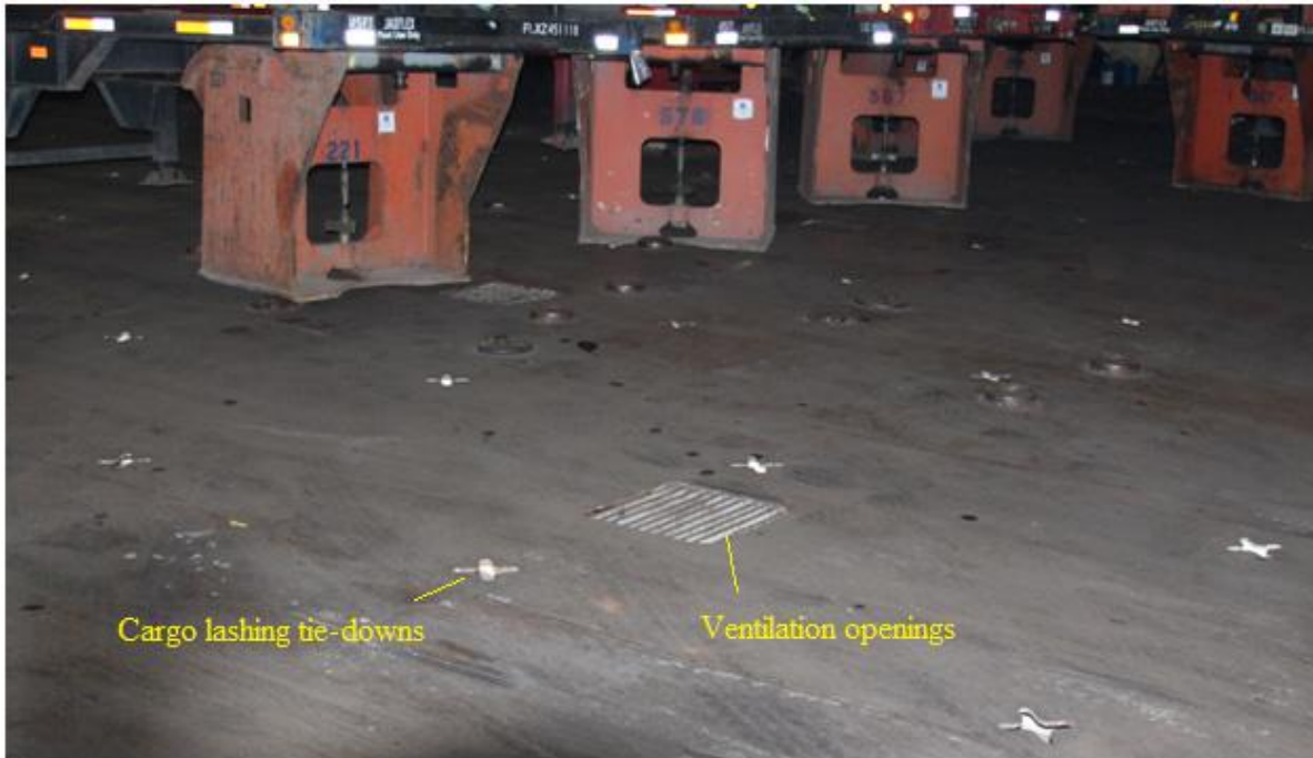
Figure 6-15: Hold 3, 3 rd deck, showing non-watertight openings. Photo of sister vessel EL YUNQUE. USCG photo.
