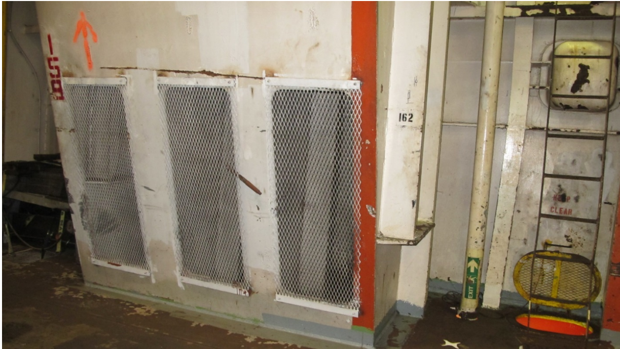
3 Tween, Stbd Side, Inlets to Exhaust Vents, Ladder up 2 nd Deck Scuttle and No. 3 hold
