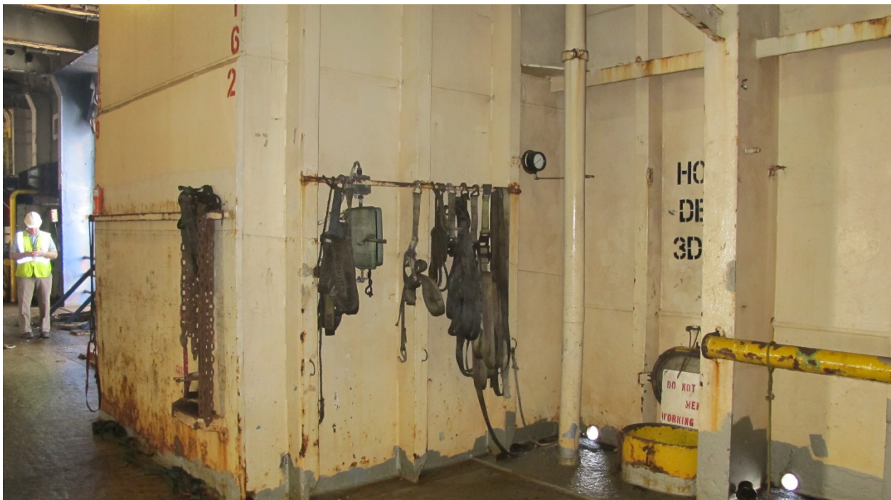
Scuttle on 2 deck, stbd side, frame 163.5 – access down to No. 3 tween and No. 3 Hold
