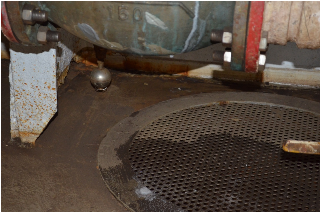
No. 3 Hold, view of rosebox cover and bilge alarm sensor, looking aft
