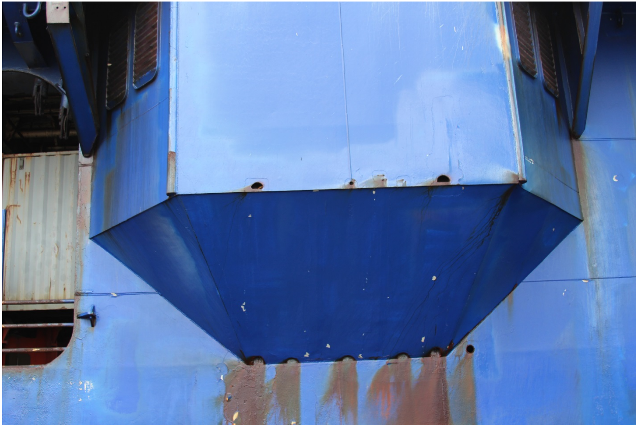
Stbd Side Inlet Vent blister, frame 142
