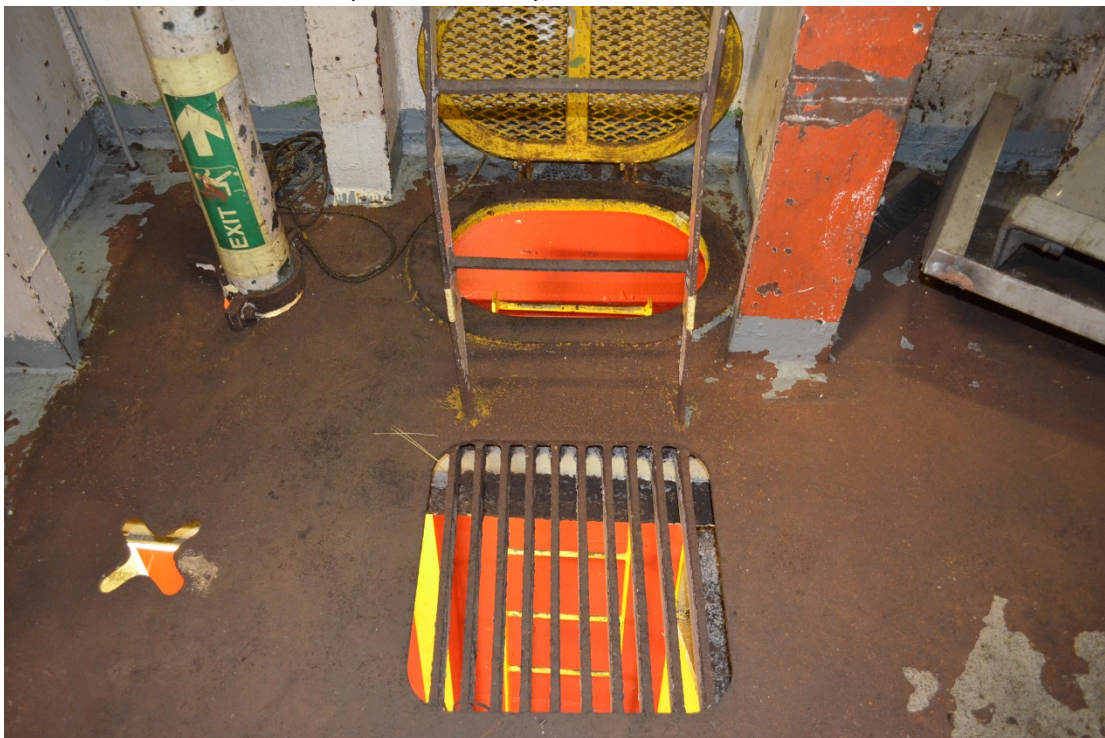
3 Tween, Stbd Side, 3 rd Deck (x-holes in deck), ladder down to No. 3 hold
