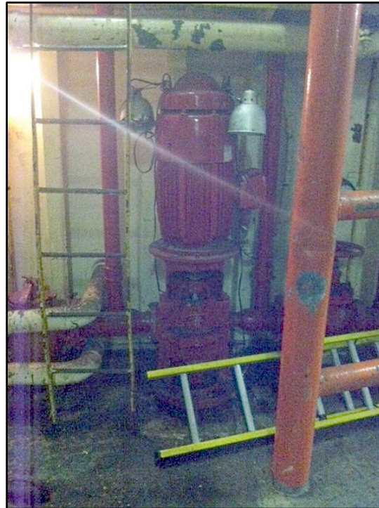
6 7 Figure 15. El Faro emergency fire pump, located at starboard frame 164, viewed from tanktop 8 deck looking aft. (Photo by Maine Maritime Academy cadet, 2015)
