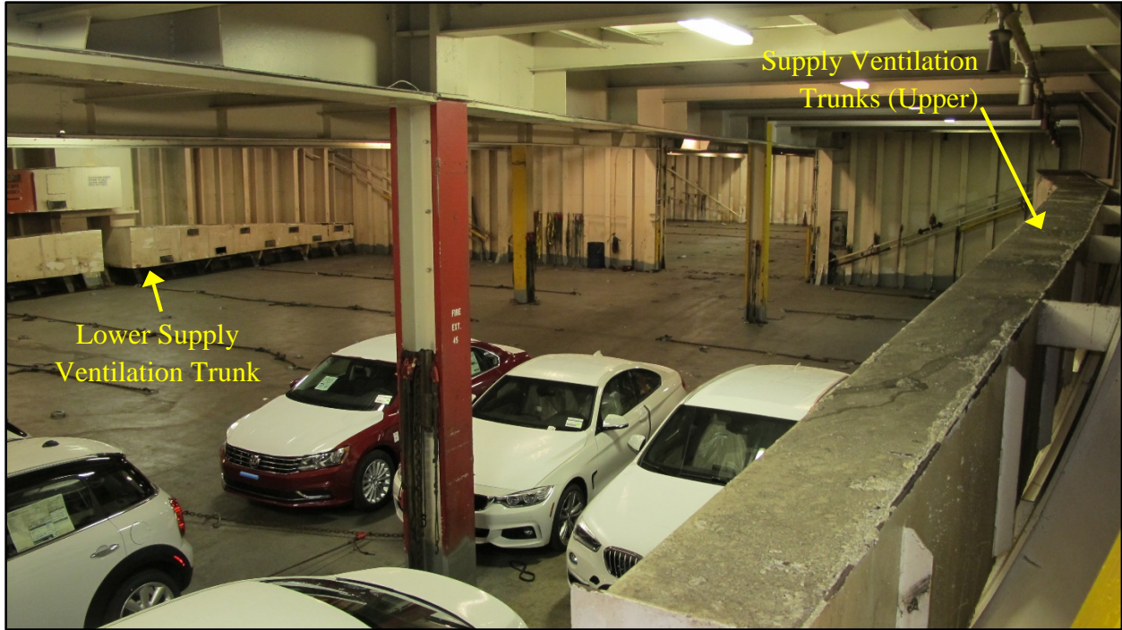
1 2 Figure 28. El Yunque , view of hold 3 from vertical ladder at frame 163.5, looking forward. (Photo 3 from December 2015)
