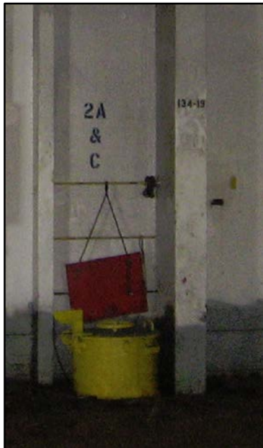
4 5 Figure 12. El Faro second deck scuttle to hold 2A, port side at frame 134-19.5. Scuttle type similar 6 to hold 3 scuttle in Figure 11. (HEC photo, July 2015)
