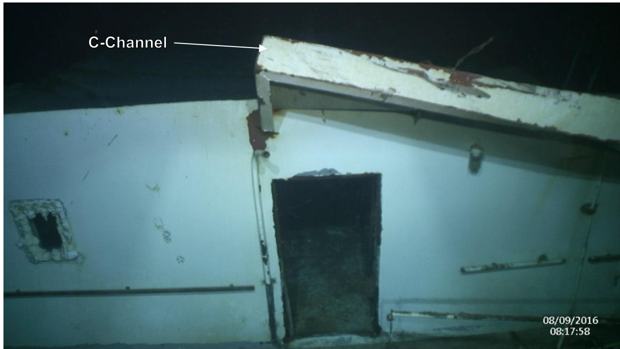
Figure 118. Region: Deck House – AFT Source: Mission III Vehicle: CURV 21
