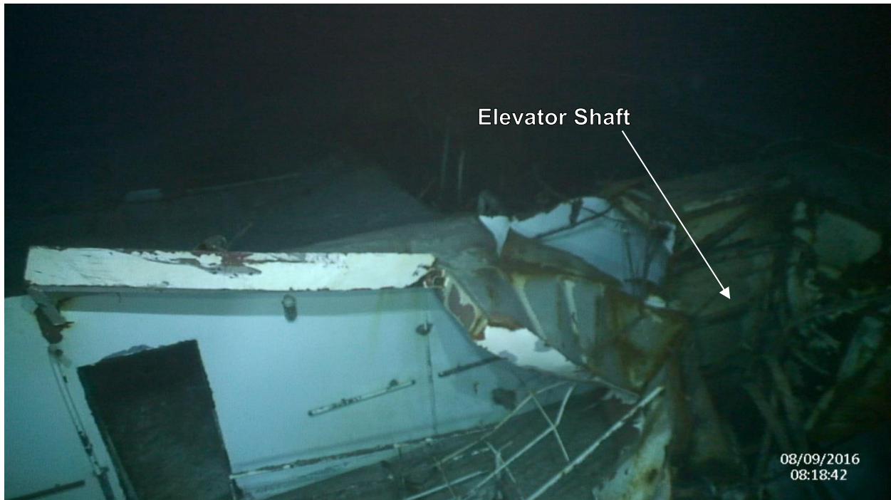
Figure 120. Region: Deck House – AFT Source: Mission III Vehicle: CURV 21
