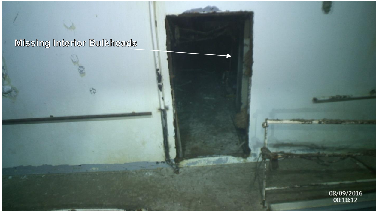
Figure 119. Region: Deck House – AFT Source: Mission III Vehicle: CURV 21
