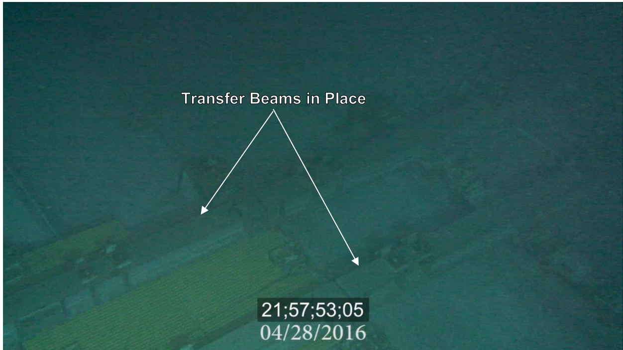
Figure 102. Region: Main Deck (forward) – Bay 14 and 15 Source: Mission II Vehicle: AOV
