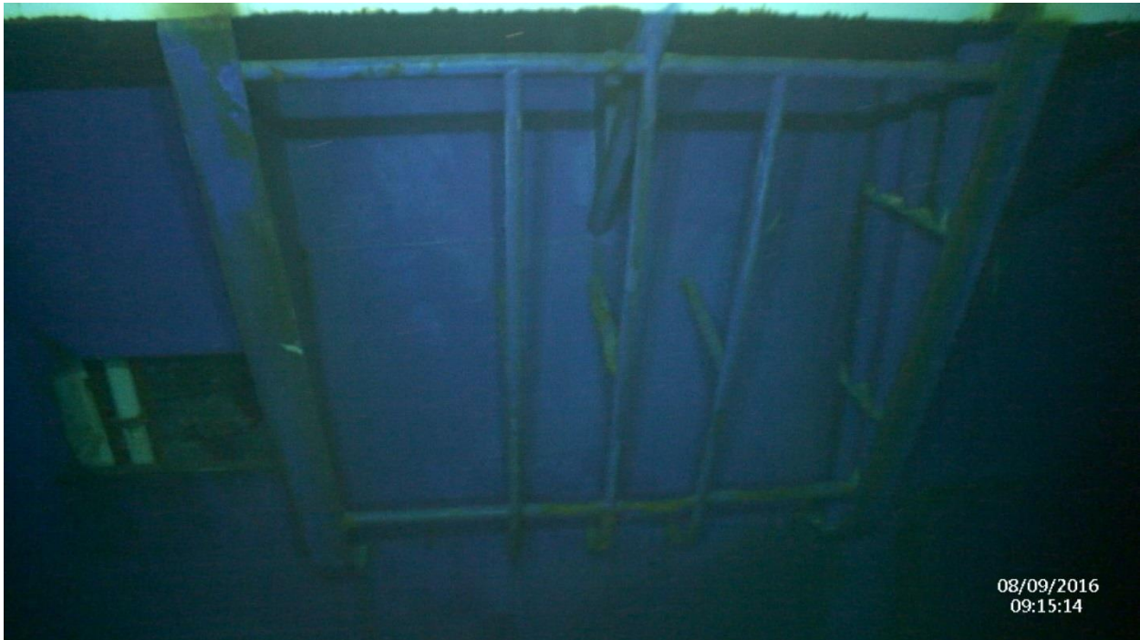
Figure 74. Region: Starboard – Life Boat Skid Source: Mission III Vehicle: CURV 21
